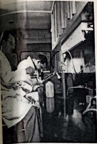
Kem-Tech Laboratory, Baton Rouge, sends truck out to make pollution surveys with equipment which includes polarized light microscope, pH meters, a 3000-watt generator, spectrophotometer, dry test meters, meteorological instruments
