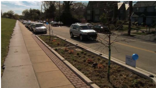
(Source: PennDOT Local Technical Assistance Program)
