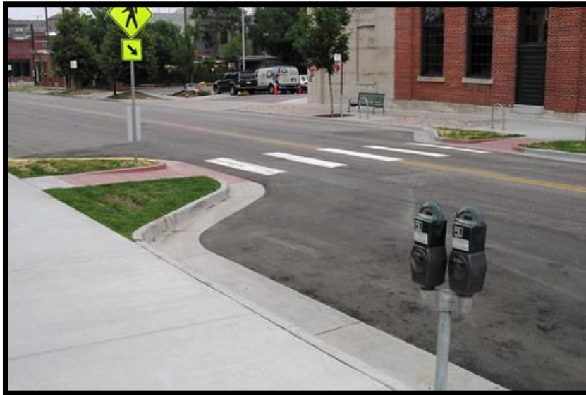
Figure 4: Sidewalk Bump Outs
