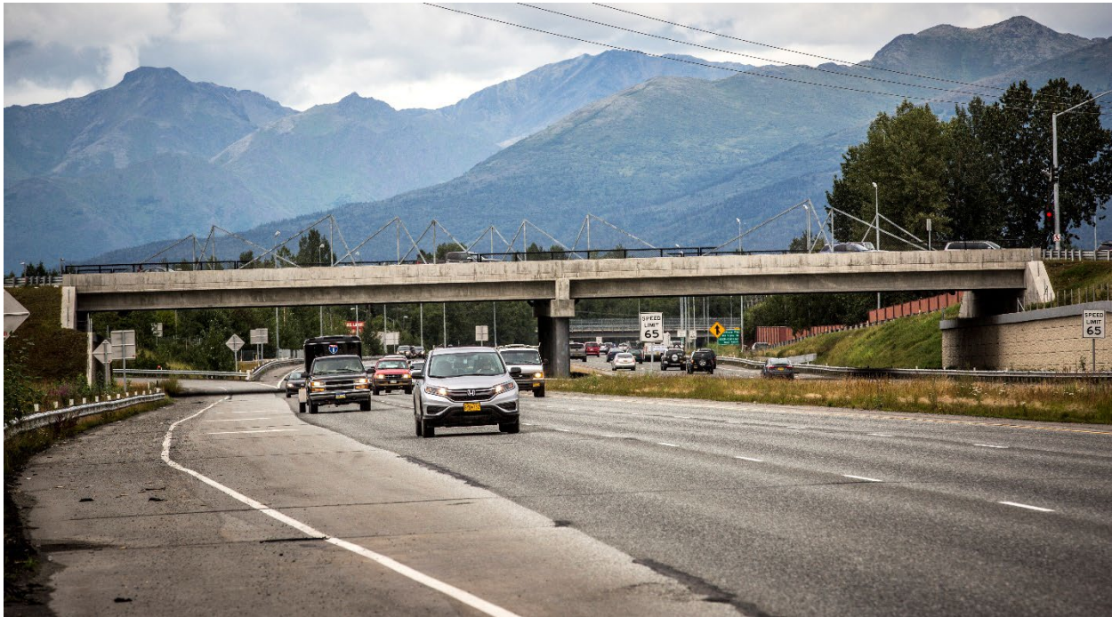
Figure 2. Freeway Example – Glenn Highway, Anchorage
