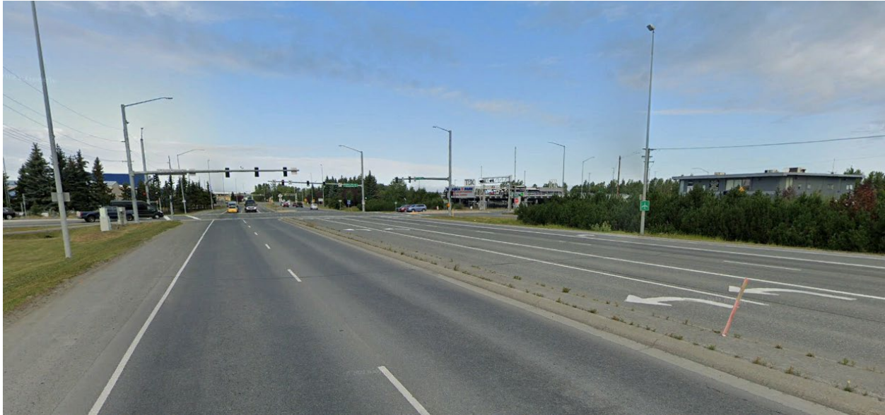
Figure 3. Expressway Example –International Airport Road, Anchorage
