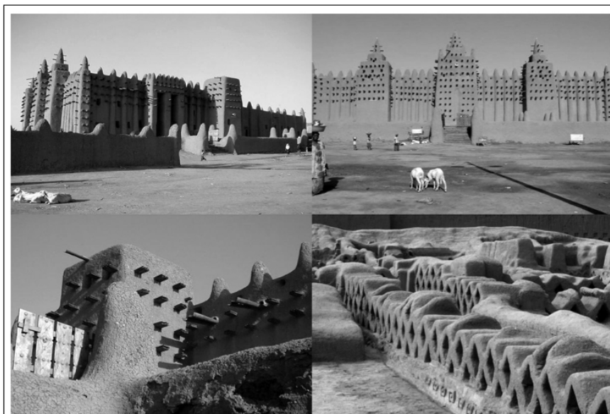
Figure 3.11: The Great Mosque of Djenné is the largest mud-brick (or adobe building) in the world and is considered by many architects to be one of the greatest achievements of the Sudano-Sahelian architectural style, with Islamic influences. Source: http://en.wikipedia.org/wiki/Great_Mosque_of_Djenné
