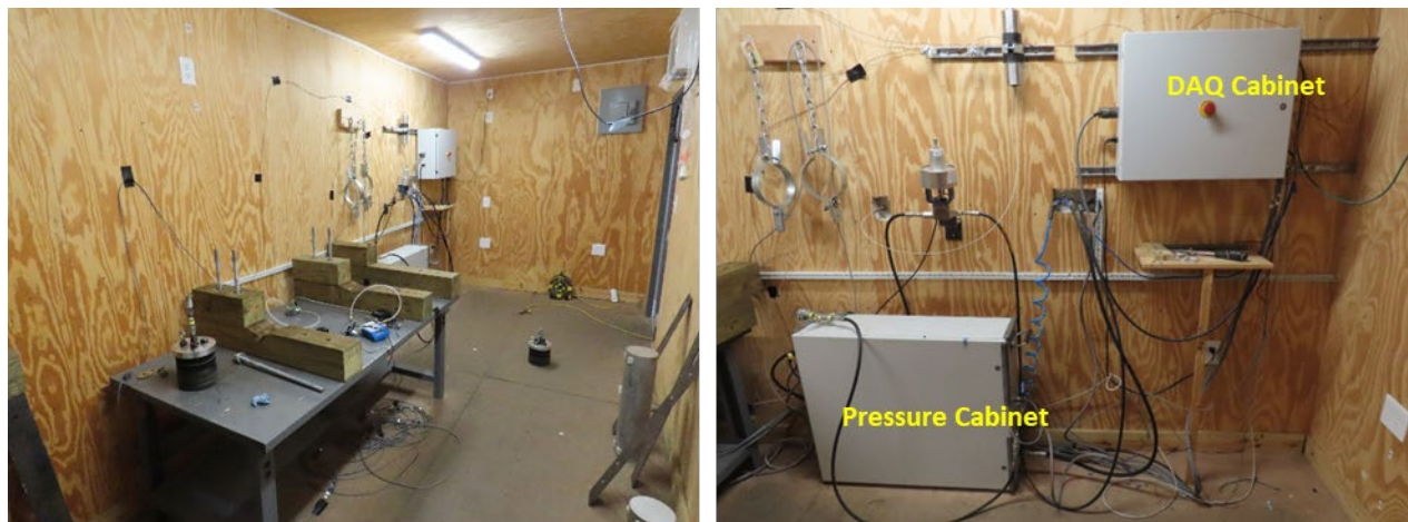
Figure 143: Interior Views of the Leak Test Structure
