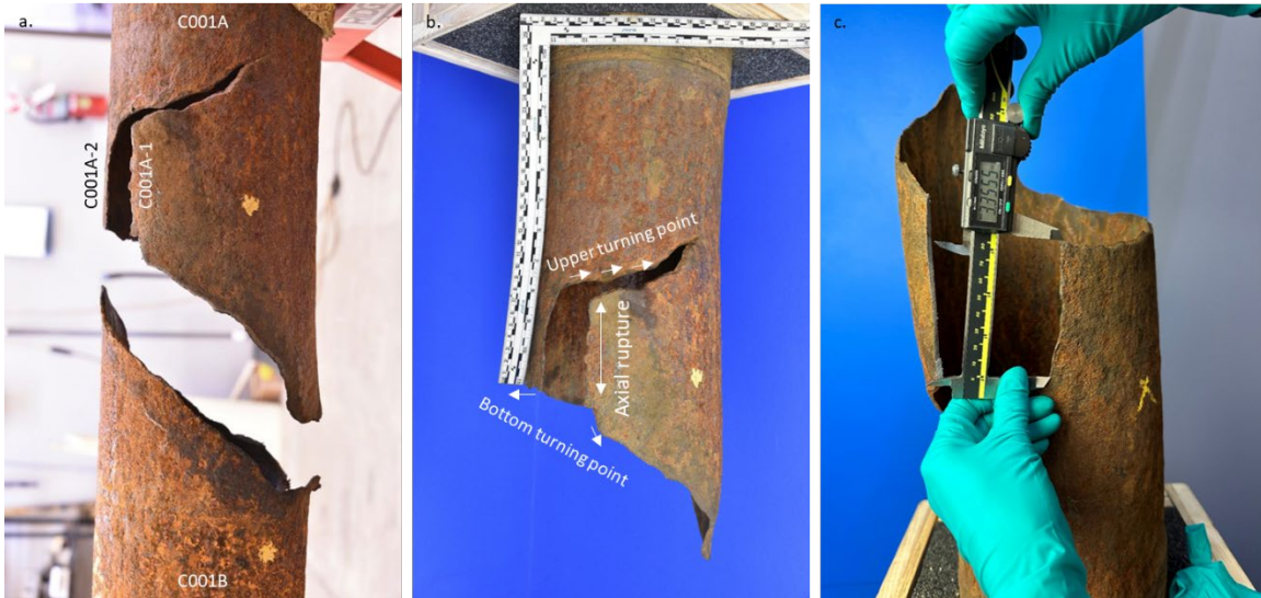
Figure 29: (a) C001B and C001A Fracture Fragments Showing Location of Axial Rupture in C001A, (b) Crack Direction in Axial Rupture, and (c) Measurement of Axial Rupture Length
