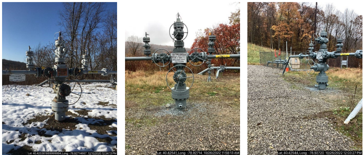
Figure 161: Well #2248 December 10, 2020, Left; October 26, 2023, Middle and Right [DEP]
