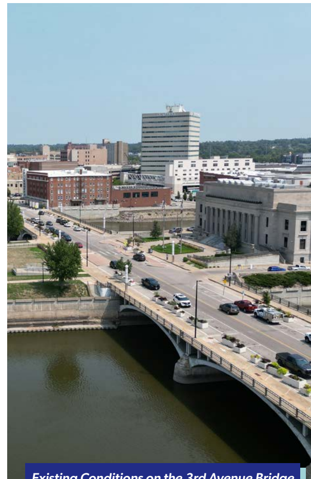
Existing Conditions on the 3rd Avenue Bridge
