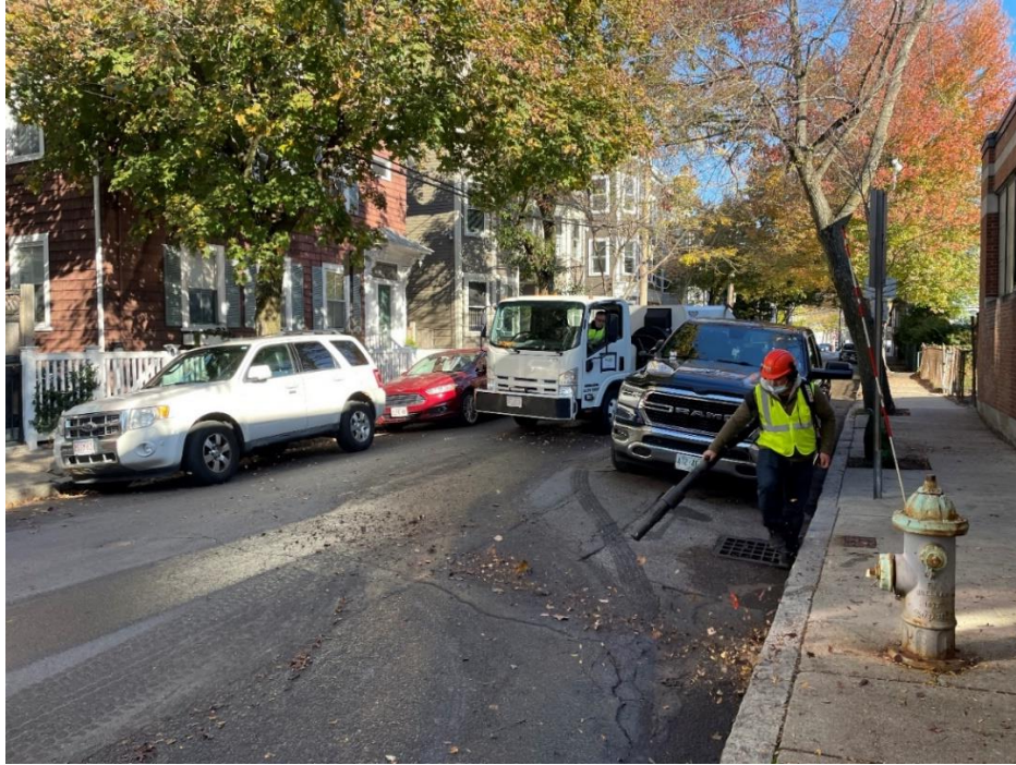
Photo Above: Hand Crews continue to clear leaves and debris from underneath a parked vehicle and an adjacent catch basin.
