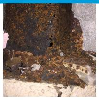
**Artifact 1 & 2:** Highly corroded metal beam in the concrete pillar is visibly corroded to a high degree
