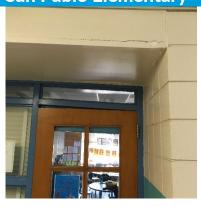
**Artifact 1:** Structural cracks are visible above the door. It is clear that the door frame is out of "square" and maintenance has been to the school to remount the classroom door to ensure it does lock and secure in case of an emergency.
