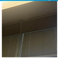
**Artifact 1:** Cracks began to form along the ceiling along the outer wall at Fishweir.
