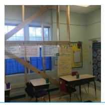
Artifacts 3, 4, 5, & 6: Pictured is the support structure that was built after engineers confirmed the sub floor could support the roof. The wing experiencing this issue was built in 1924. The original area of the school was built in 1917.
