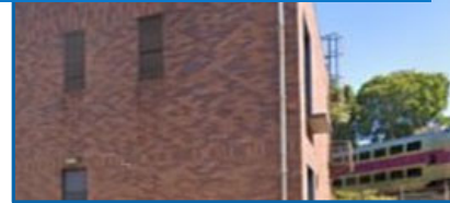
Traction Power Substation (TPSS) Equipment
