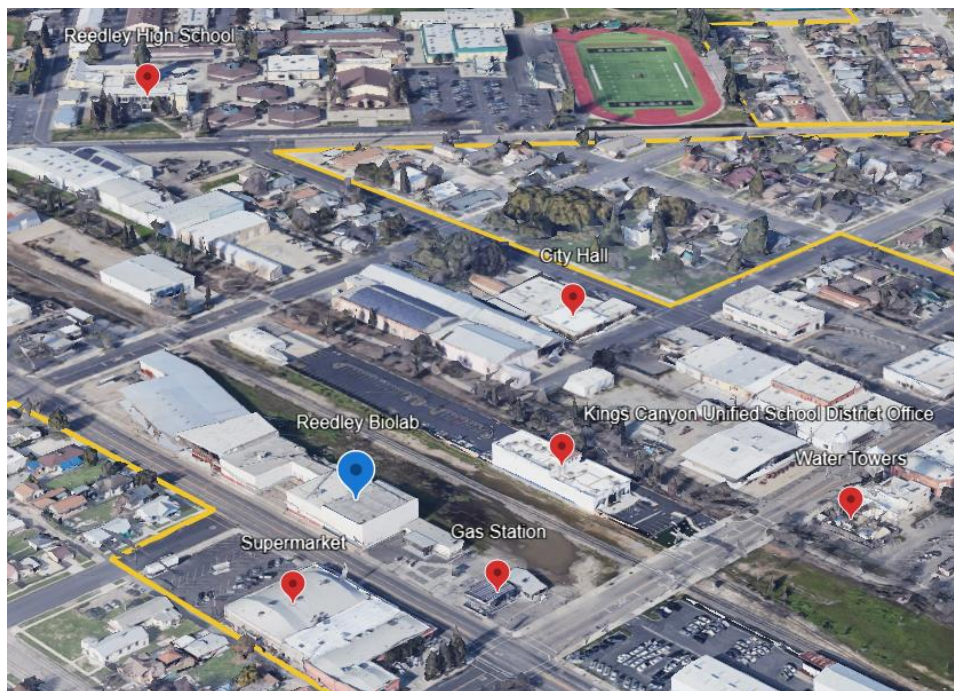
Figure 1 - Aerial view of Reedley, with Reedley Biolab in blue, major landmarks in red, and residential areas in yellow. Source: Google Earth.
