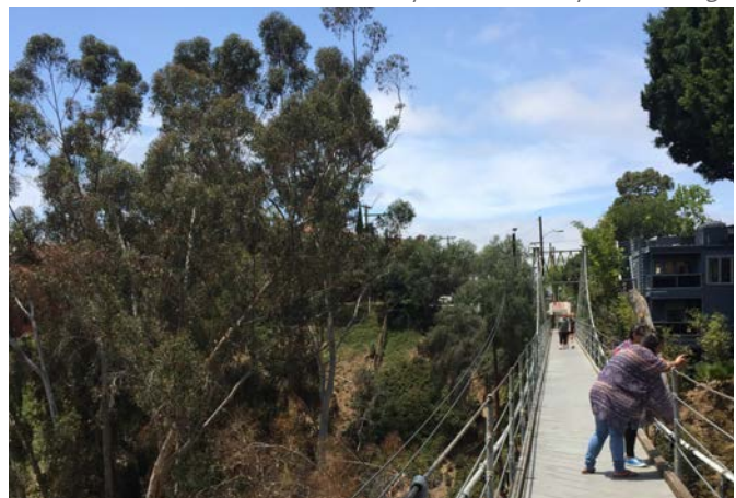
Spruce Street Suspension Bridge
