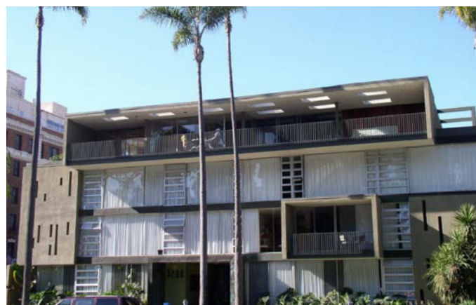
The Colonel Irving Salomon/Henry Hester Apartments, completed in 1958, was originally commissioned as a luxury apartment building.
