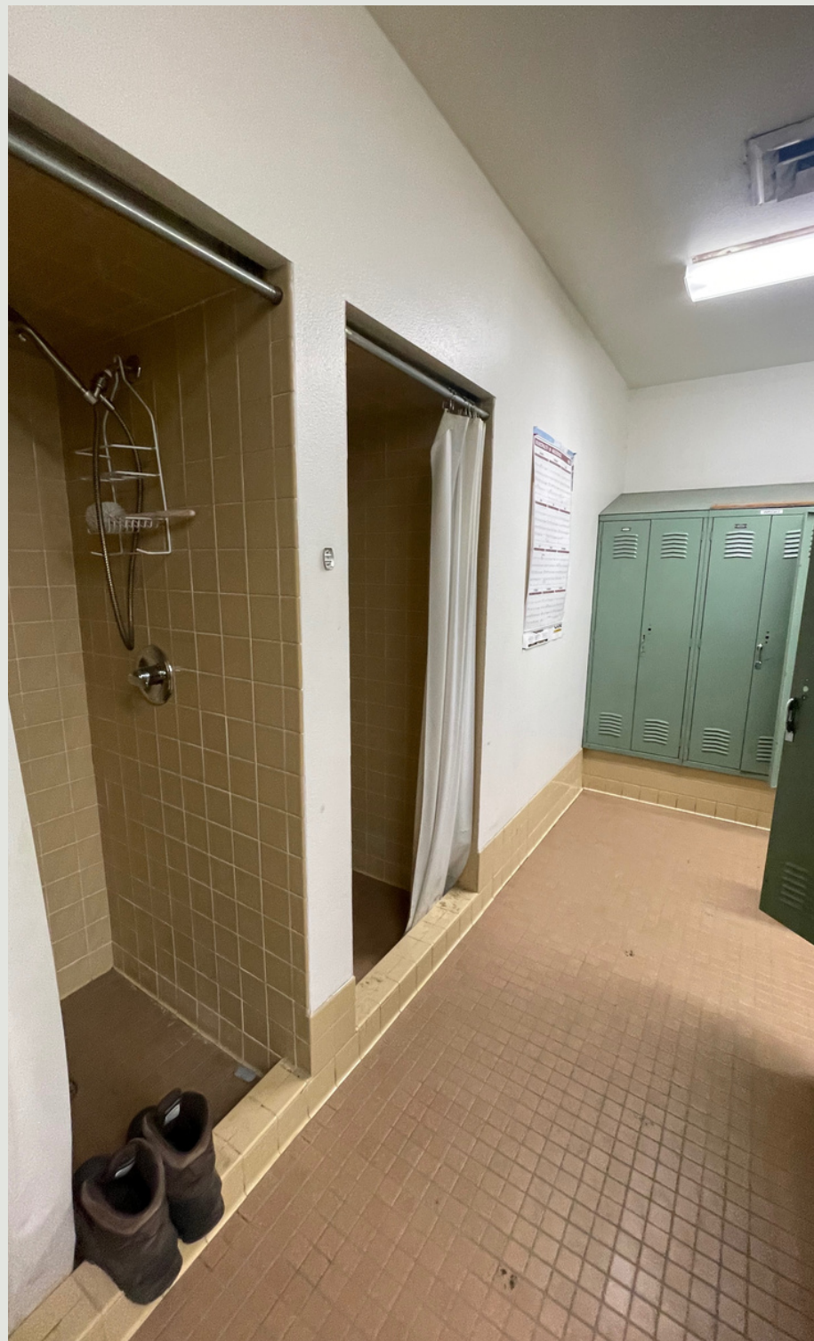
Men & Women's Bathrooms are fully functional, 3 showers on site.
