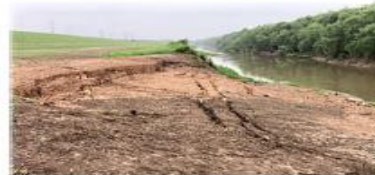
Erosion on Trinity River
