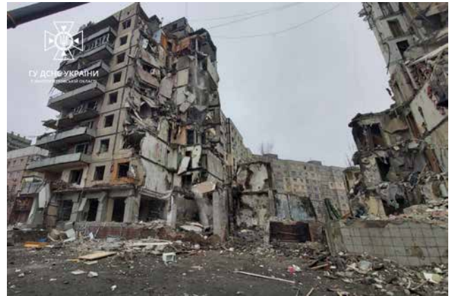
An apartment building in Dnipro, central Ukraine, that was destroyed by a Russian missile strike on January 14, 2023 (January 2023) [Facebook account of the Government of Ukraine]
