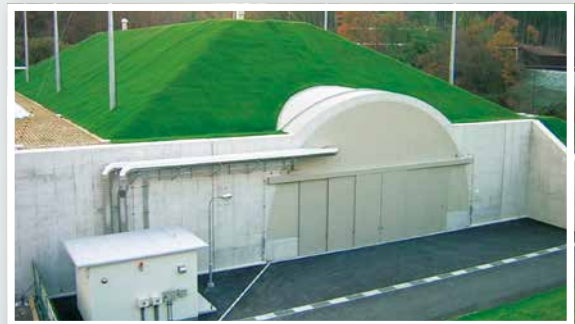
Securing ammunition storage facilities
