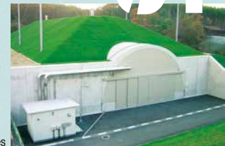
Securing ammunition storage facilities
