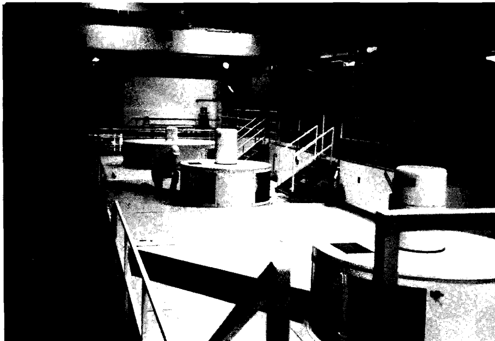
An interior view of the Snettisham Powerplant, which is the only powerplant in Alaska located underground.
