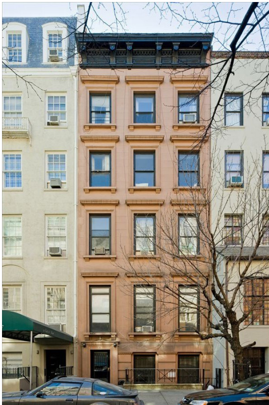
Figure 7.1 34 East 68 th Street after restoration
