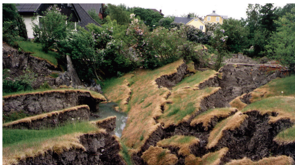
Landslide. Source: Swedish Geotechnical Institute
