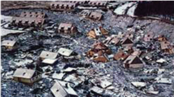
Quick clay slide. Source: Geological Survey of Sweden archives/Curt Fredén
