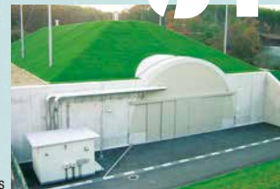
Securing ammunition storage facilities
