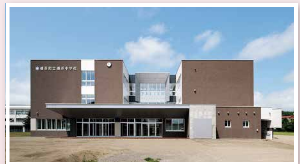
Subsidy for noise prevention work (Shibecha Junior High School, Shibecha Town, Kawakami-gun, Hokkaido)
