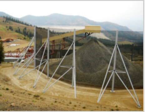
Complete Stockpile Enclosure
