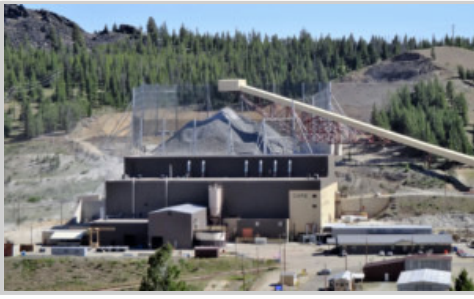
Stockpile Wind Fence
