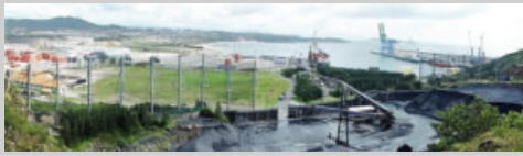
Wind Fence Port Facility
