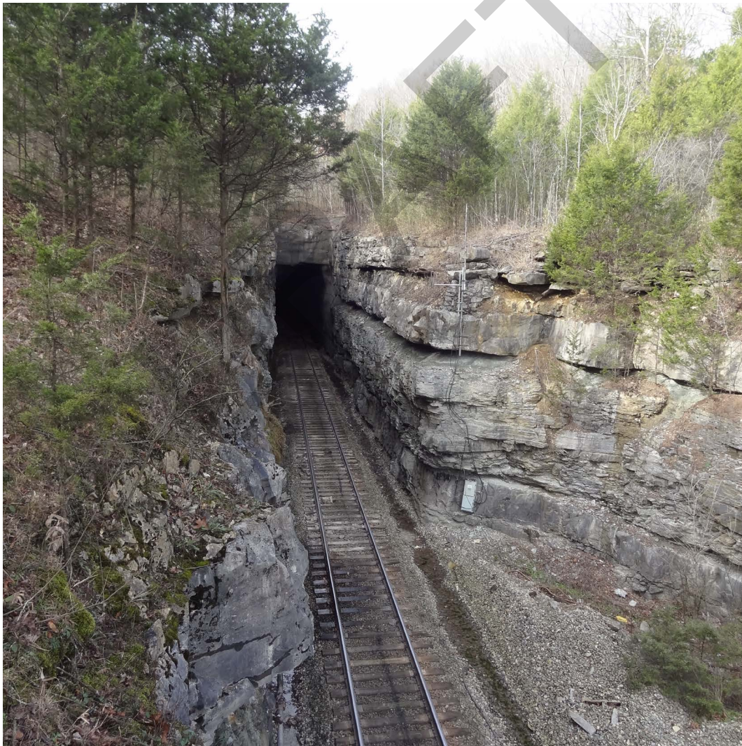
Cowan Tunnel, Franklin County, Tennessee
