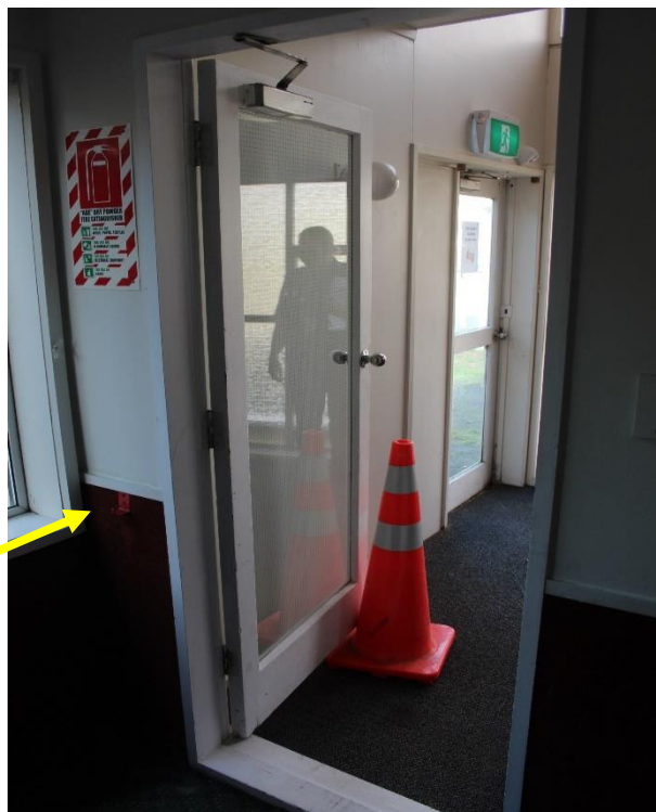
Photo 7: B Block, Ground level rear
