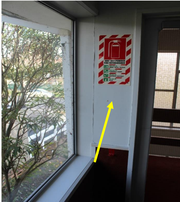
Photo 8: B Block, upper level
