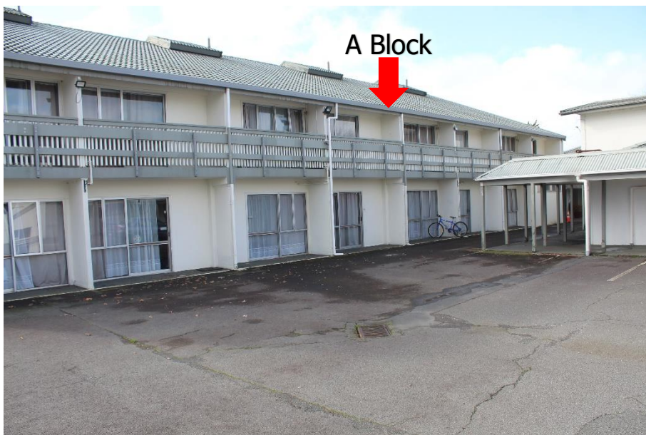
Photo 2: View of motel units 1-24
