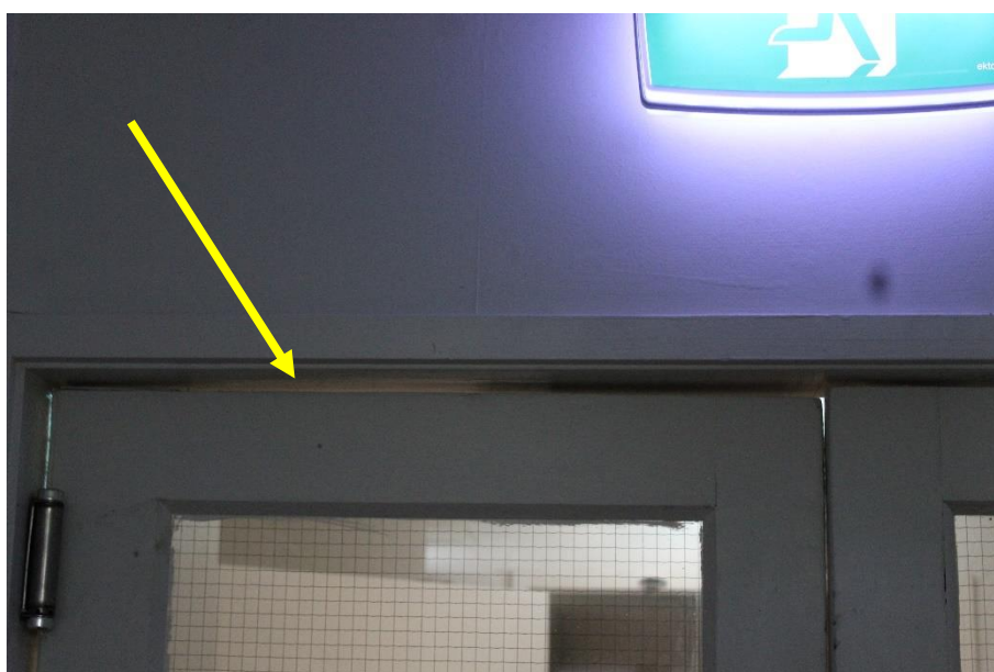
Photo 10: Close-up smoke-stop doors, A Block, upper level
