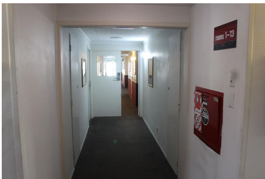
Photo 14: A Block, ground level
