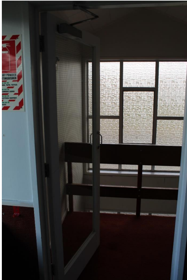
Photo 11: Smoke-stop doors, upper level
