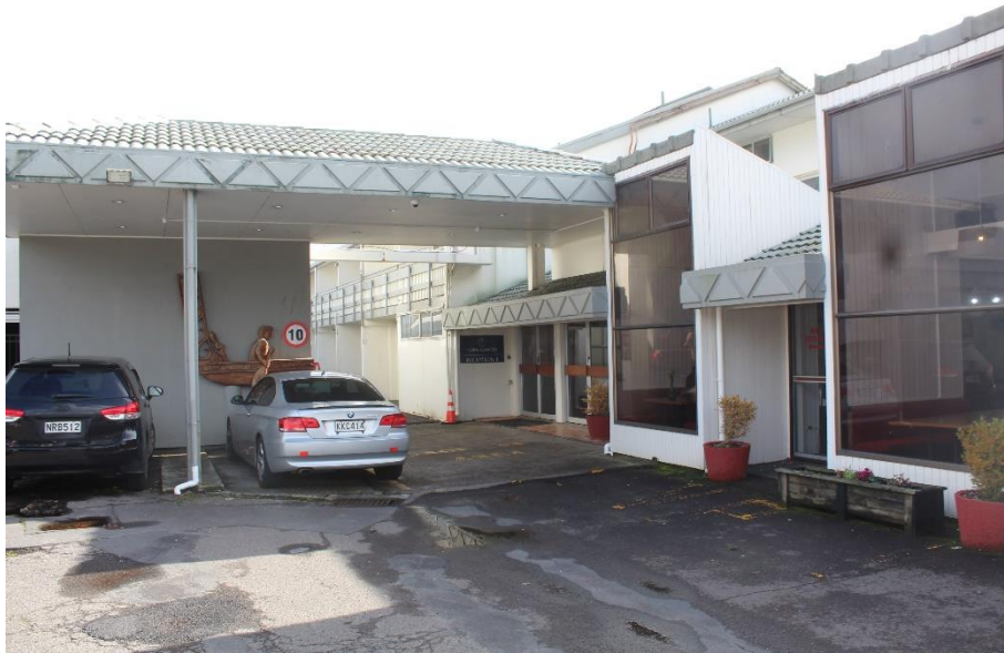
Photo 1: Front view of building
