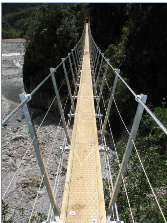
Fig. 4 Roberts Point Swingbridge, 2015
