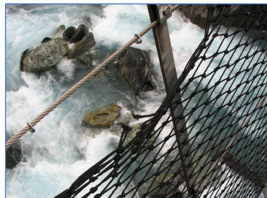
Fig. 5 Barrier-infill netting worn through at ring staples
