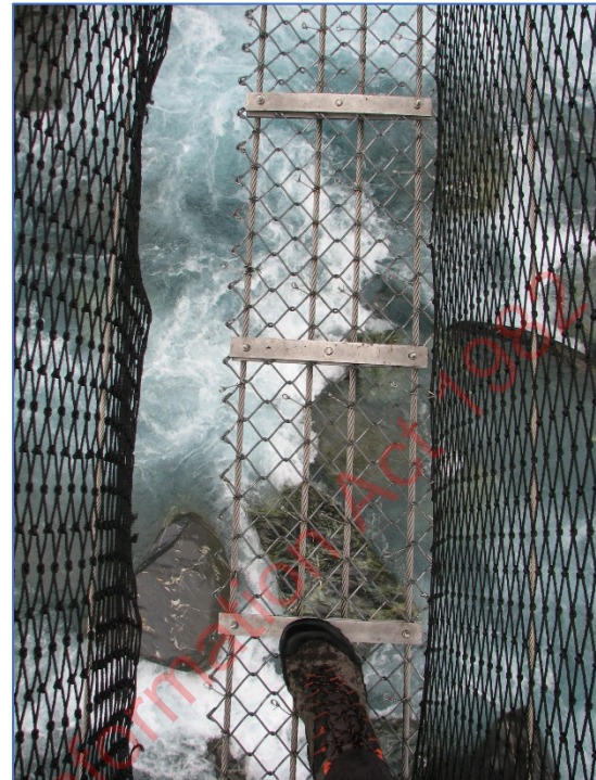
Fig. 1 Detached barrier-infill netting where the fall occurred
