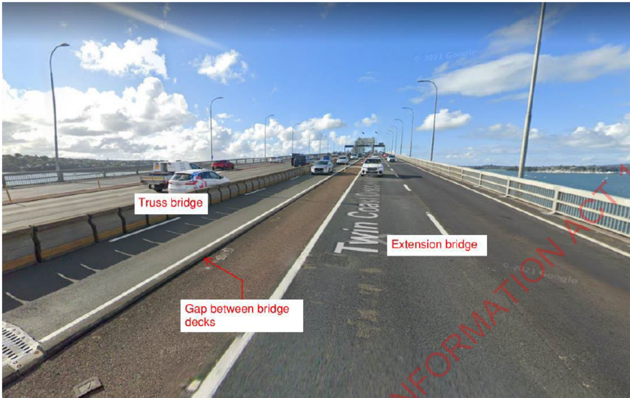
Figure 2: Gap between bridge decks
