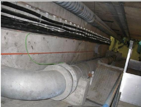
Figure 5 View inside concrete corridor
