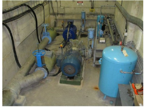
Figure 4 Intake Pump Station
