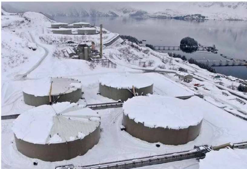
Crews work on tank top snow removal on Tanks 12 and 14 in the East Tank Farm in Valdez on March 16, 2022. (Photo provided by Alyeska Pipeline Service Co.)
