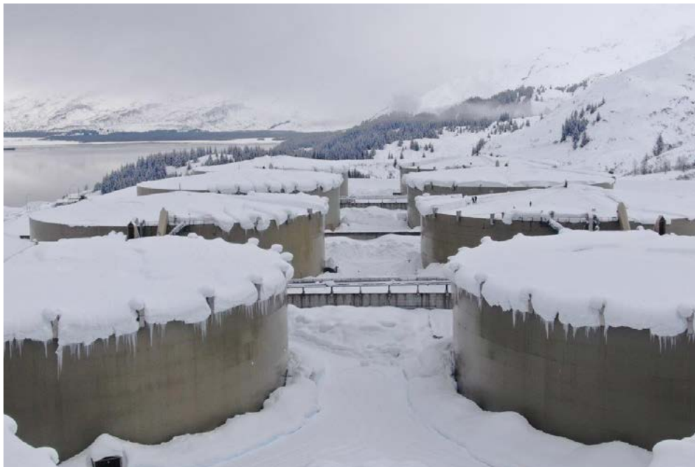
Alyeska East Tank Farm, March 2022
