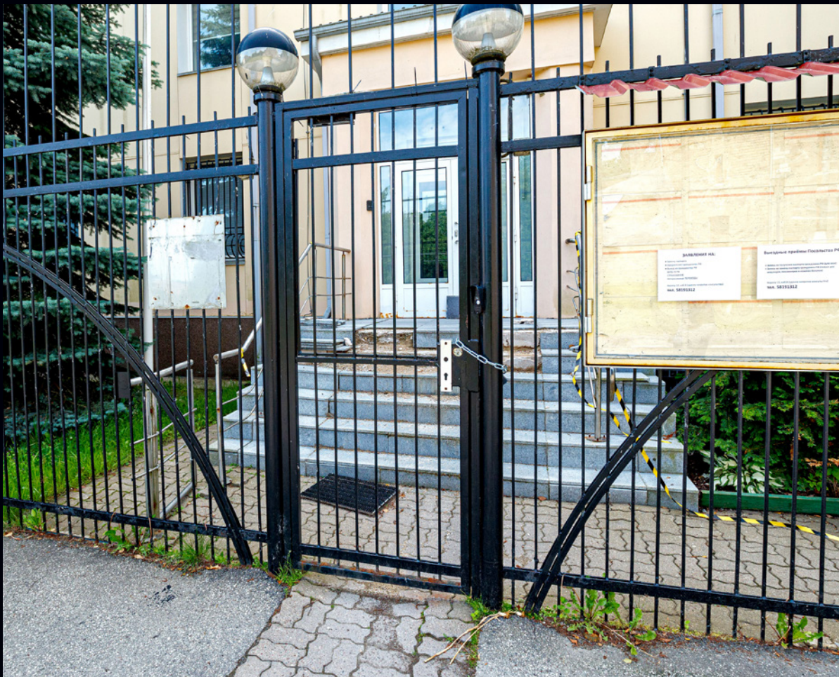
The building of the Consulate General of the Russian Federation in Narva in mid-summer 2022 Photo: Taavi Sepp, Postimees
