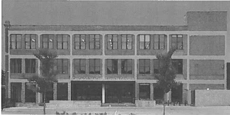
1901 W. Carroll Ave. on the Near West Side, near the intersection of Damen and Carroll.
