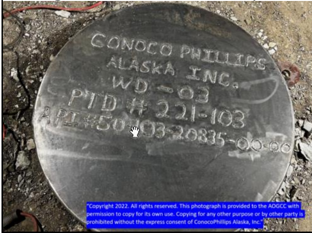
Plate Welded on WD-03, Plug & Abandonment Complete
