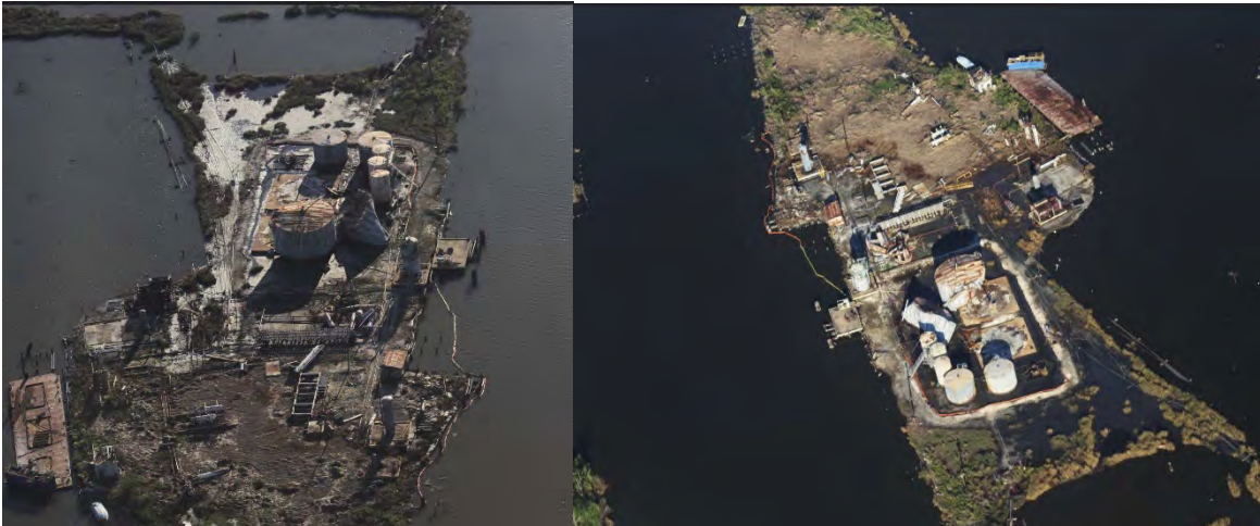
Figures 8 a and b. photos of damage to an oil and gas facility baywards of the LNG site during the passage of Hurricane Ida.
