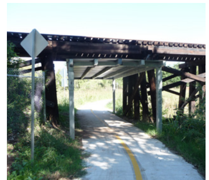
Underpass along the Southern Walnut Creek Trail
