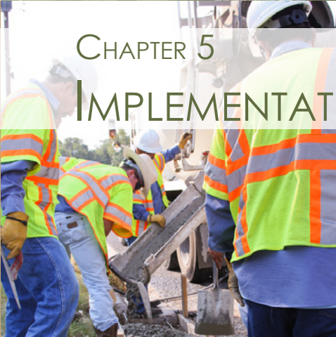
City of Austin Concrete & Asphalt Crew
