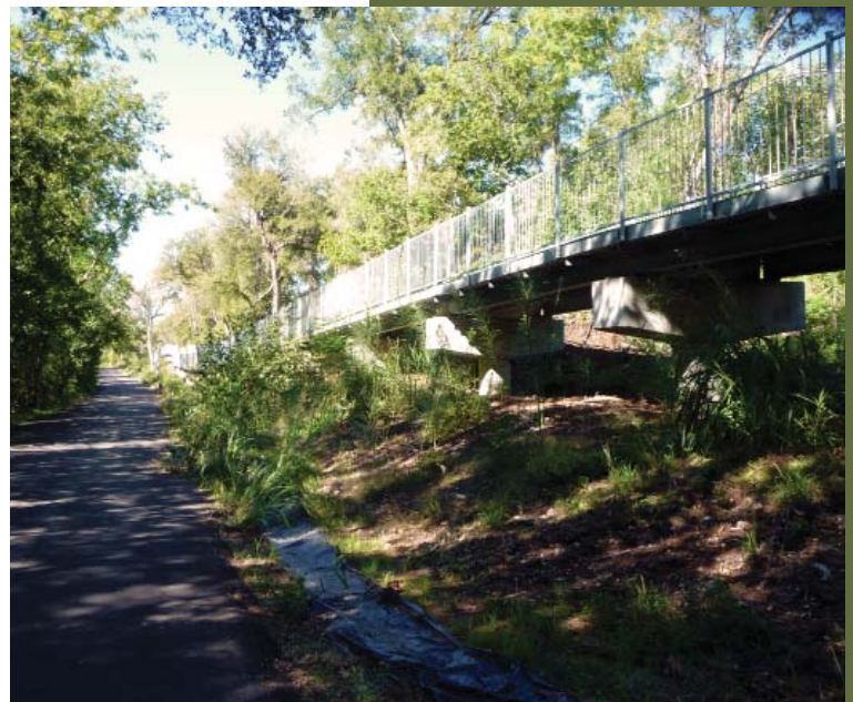
Elevated segment of the Southern Walnut Creek Trail along Delwau Lane.
