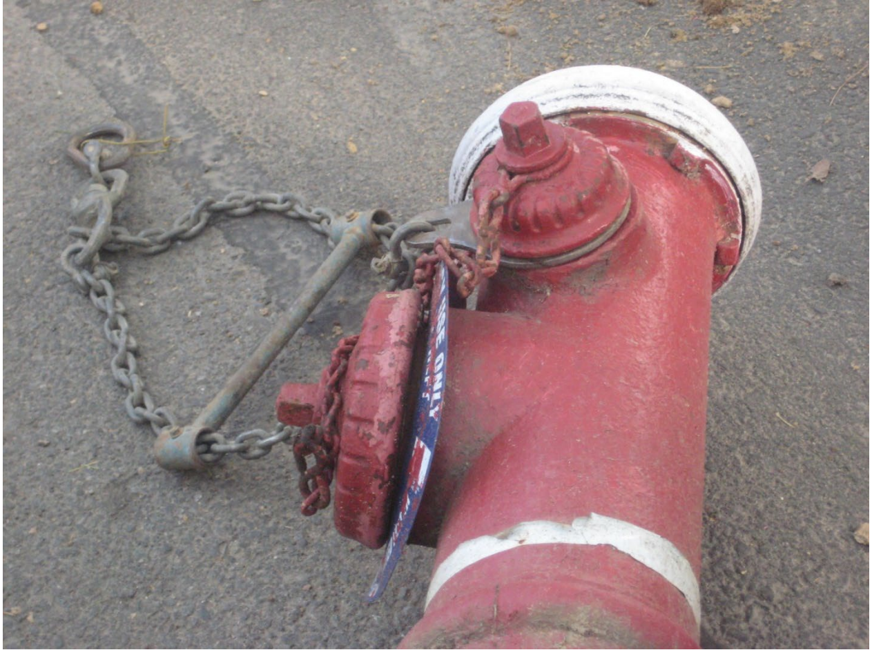
Hydrant 1-119 – Extracted Hydrant Connection Detail – April 30, 2021
