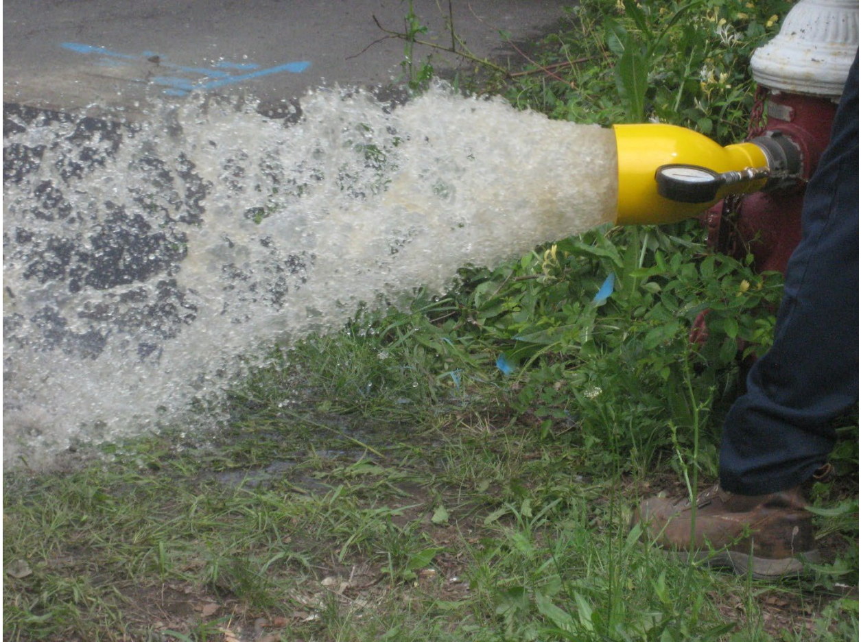
Hydrant 1-89 Flow Test – Water Consumption Demonstration – June 10, 2021
