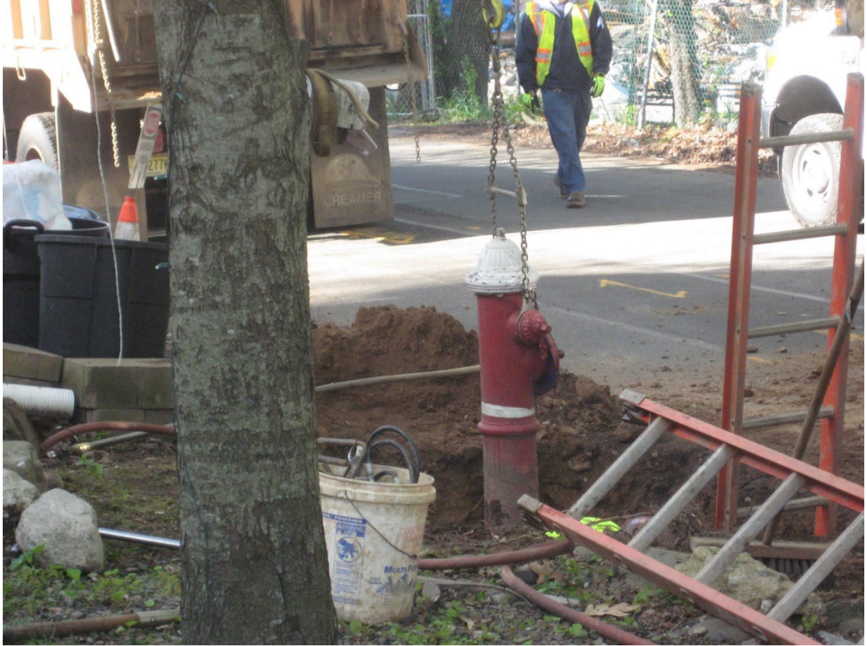
Hydrant 1-119 – Backhoe lifting hydrant for extraction – April 30, 2021
