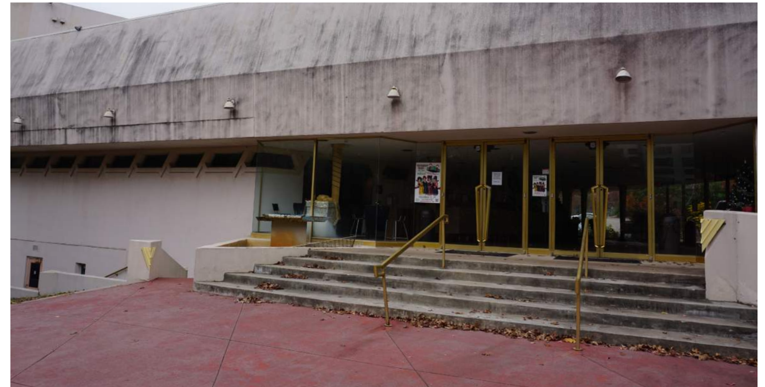
South entry existing condition
