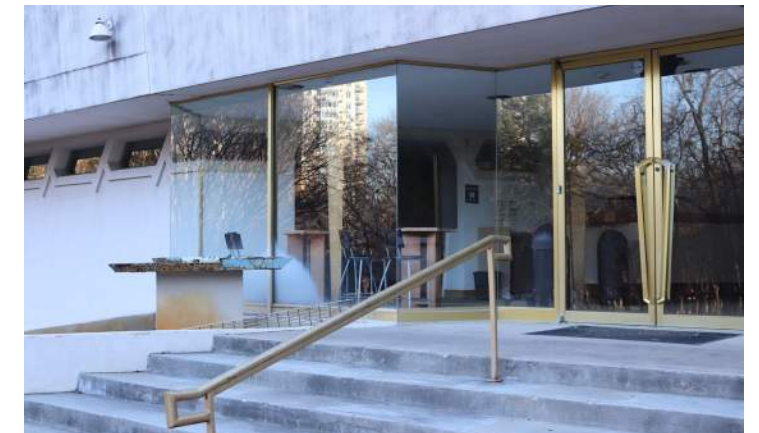
The non-original south entry paving, handrails, and fountain are in fair to poor condition.
