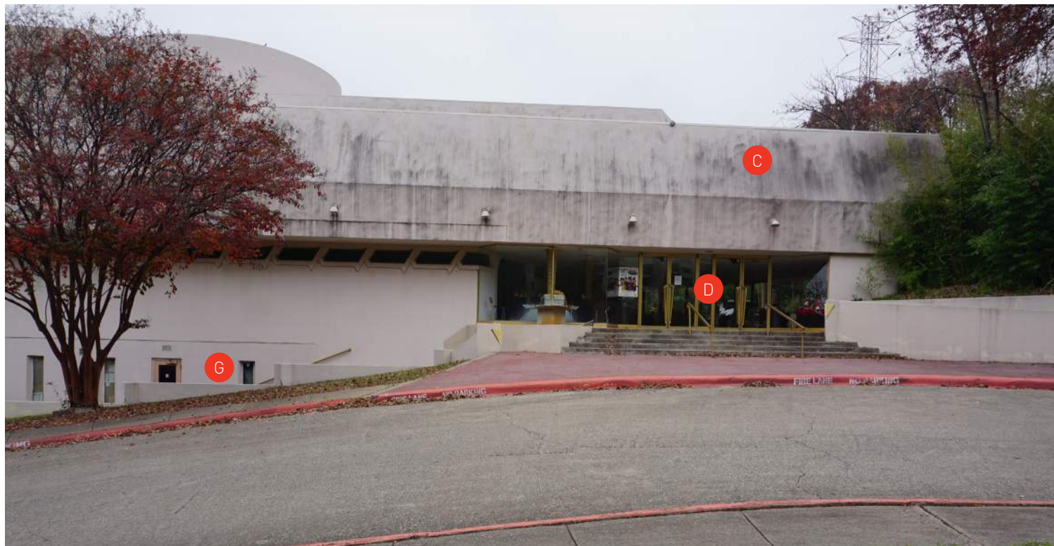
Non-original entry, education wing, and basement offices to be removed
