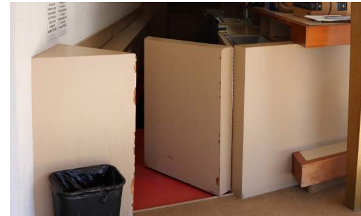
Laminate finishes on refreshment bar and red vinyl tile floor behind the counter.
