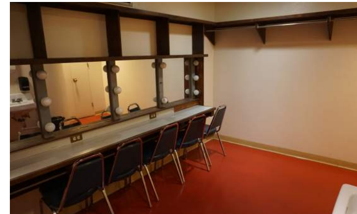
Typical condition of back of house dressing rooms
