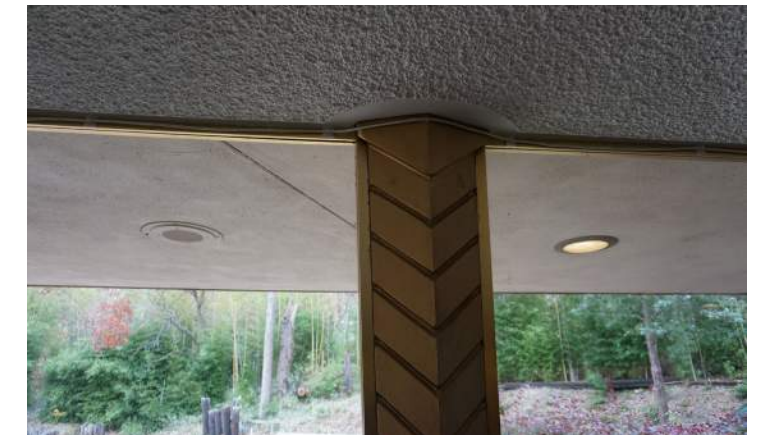
Detail of non-original glass storefront meeting ceiling and columns.
