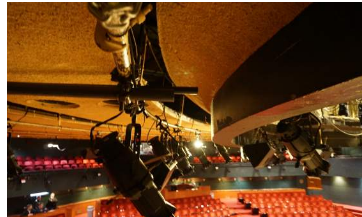
Detail of existing ceiling.
