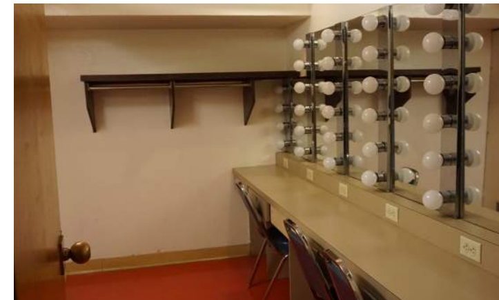
Condition of dressing rooms with non-original built ins.
