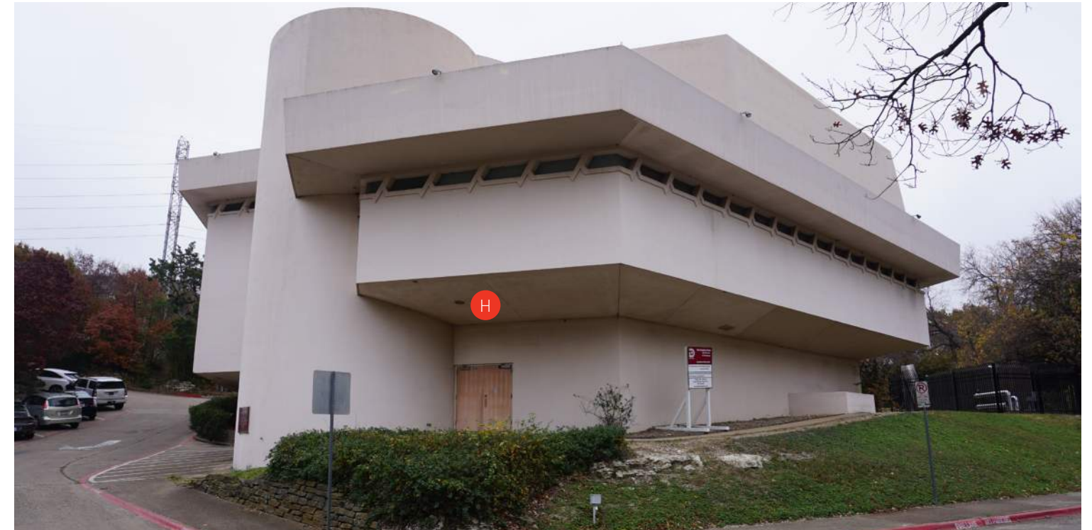
Remove existing soffits to accommodate required structural work.
