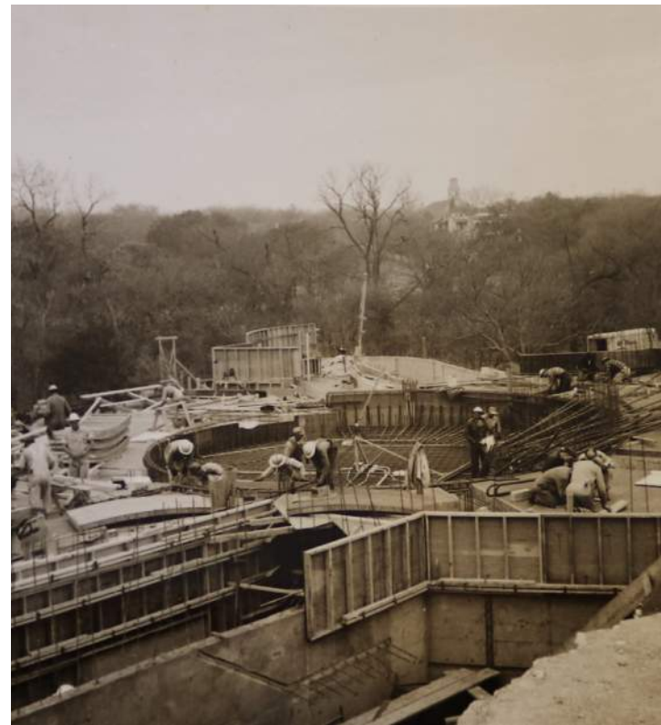
Image 4 Construction of original dropped floor stage, courtesy of DTC Theater Archives
