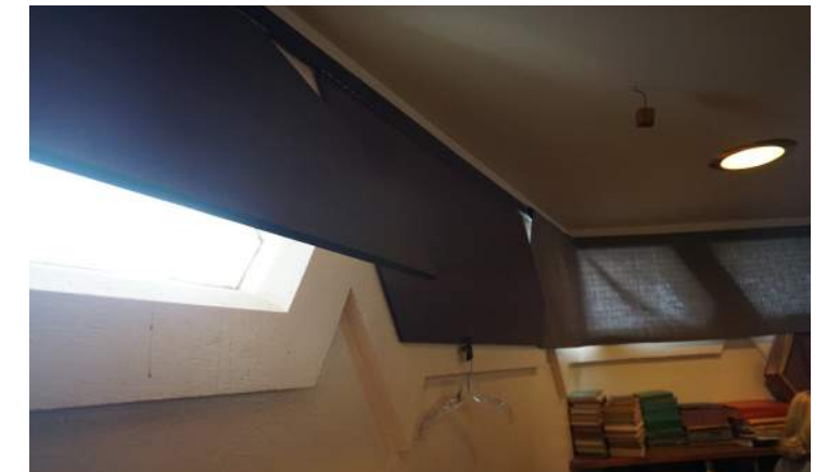
Plywood panels over four windows, fabric curtain over others.
