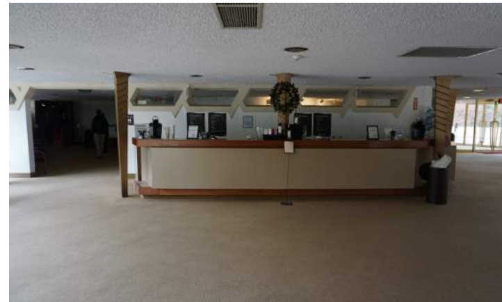
Non-original refreshment bar and opening in original concrete wall.
