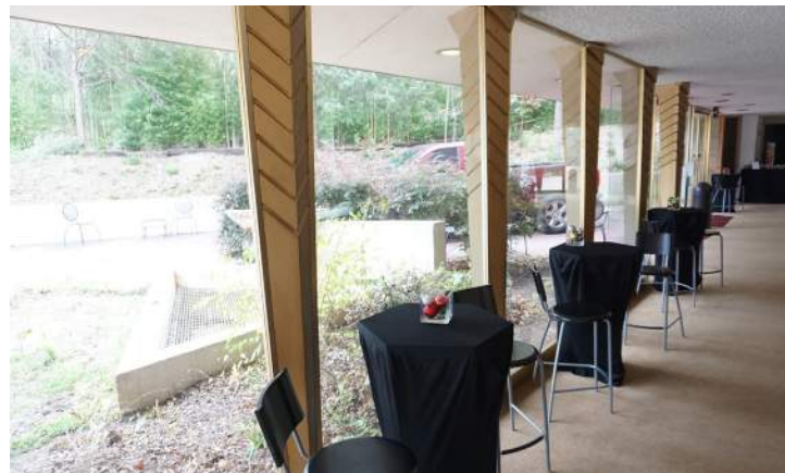
Added columns to support the education wing above.
