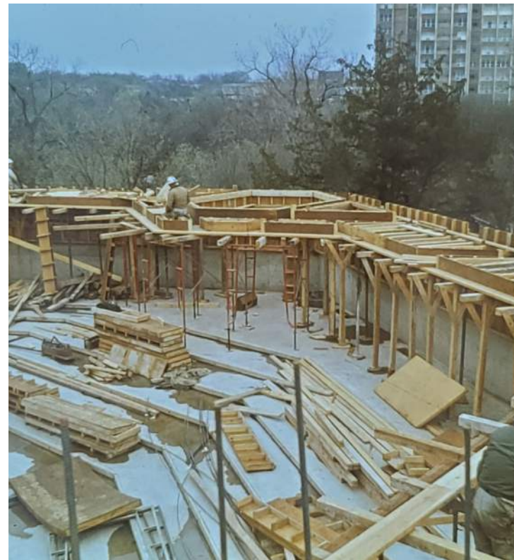
Image 22 Construction of the house balcony and installation of roof trusses
