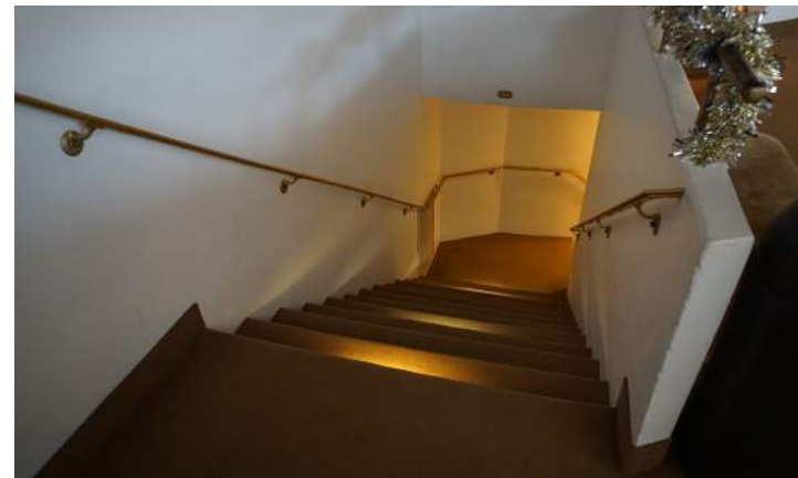
Rebuilt stairs in original location provide access to the basement level.
