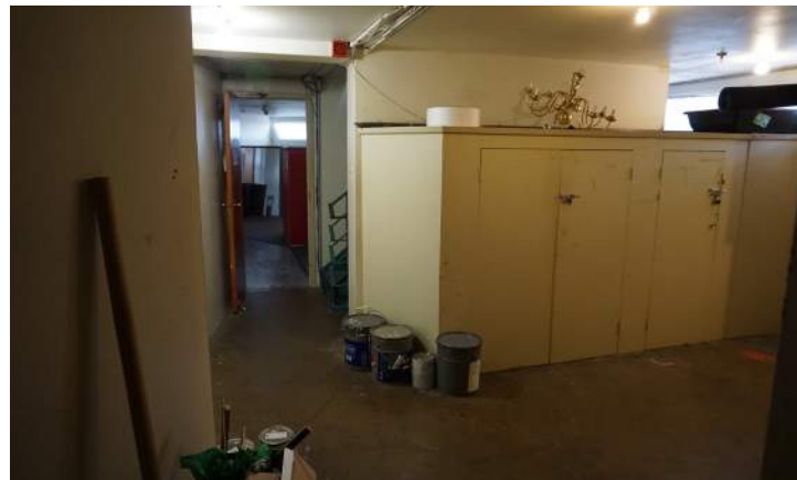
Plenum storage space.
