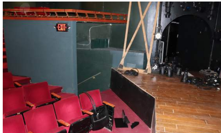
Original vomitory stairs covered for additional seating above.
