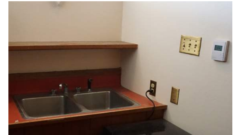
Original switch and outlet covers present throughout room.
