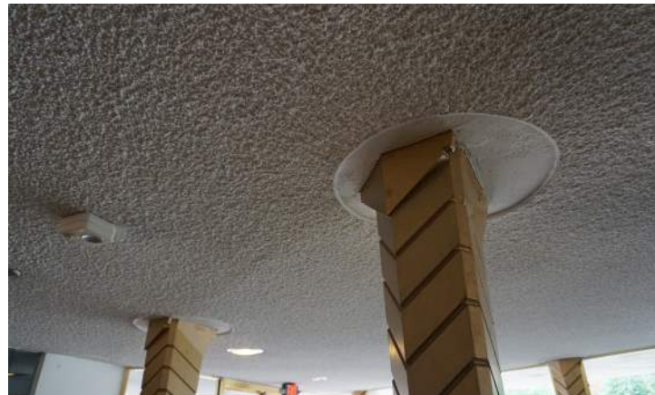
Textured plaster ceilings with smooth circles around columns.
