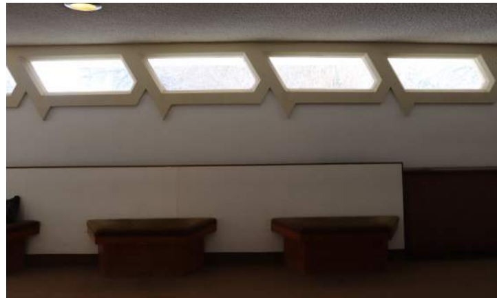
Cast concrete windows with single pane glass, typical of the building.
