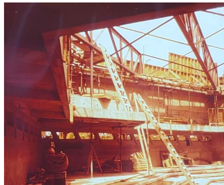
Image 23 Construction of the house balcony and installation of roof trusses
