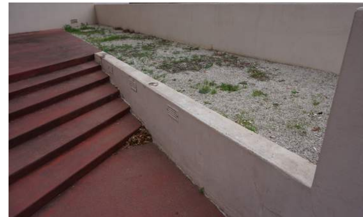
Retaining walls and planters are in fair condition.
