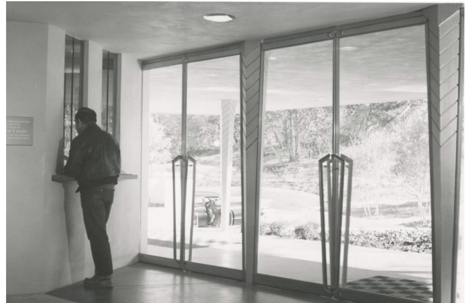
Original lobby entry condition to be restored.
