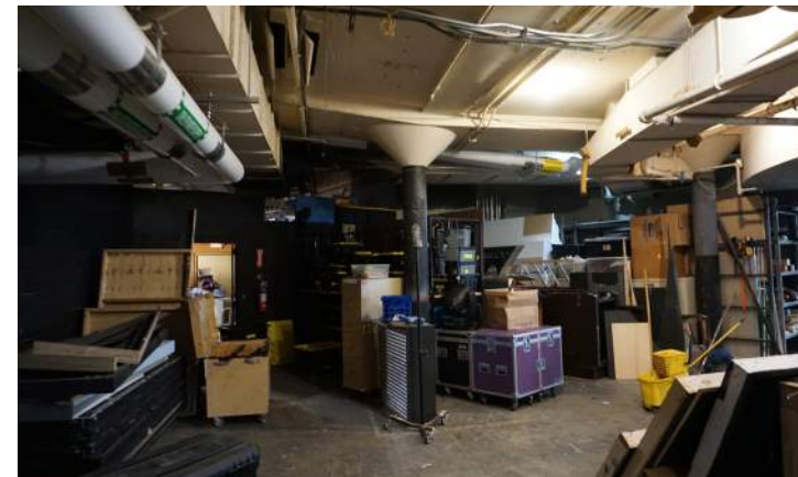
Overall view of basement workshop.
