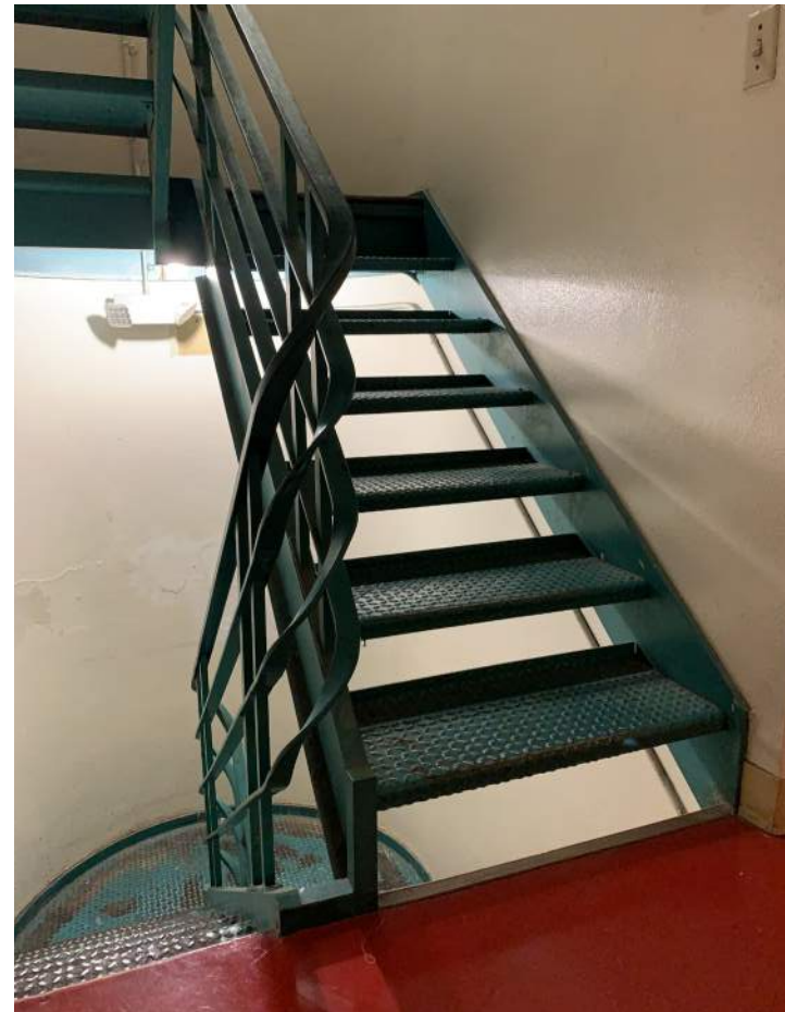
Original steel stair at back of house spaces.
