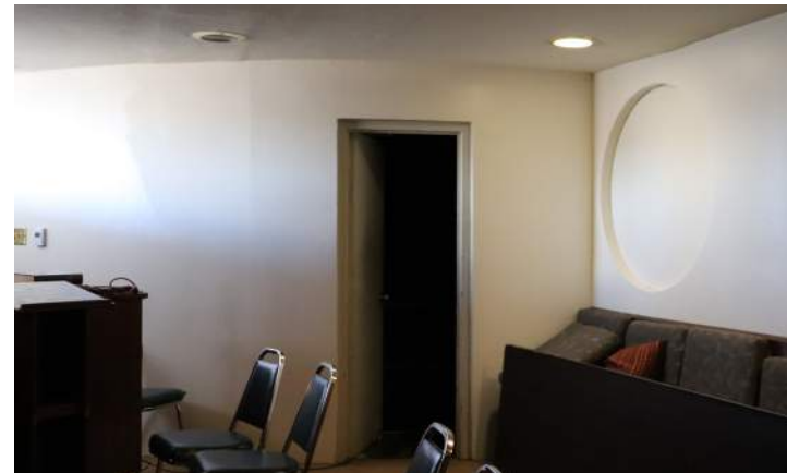
Infilled circular opening.
