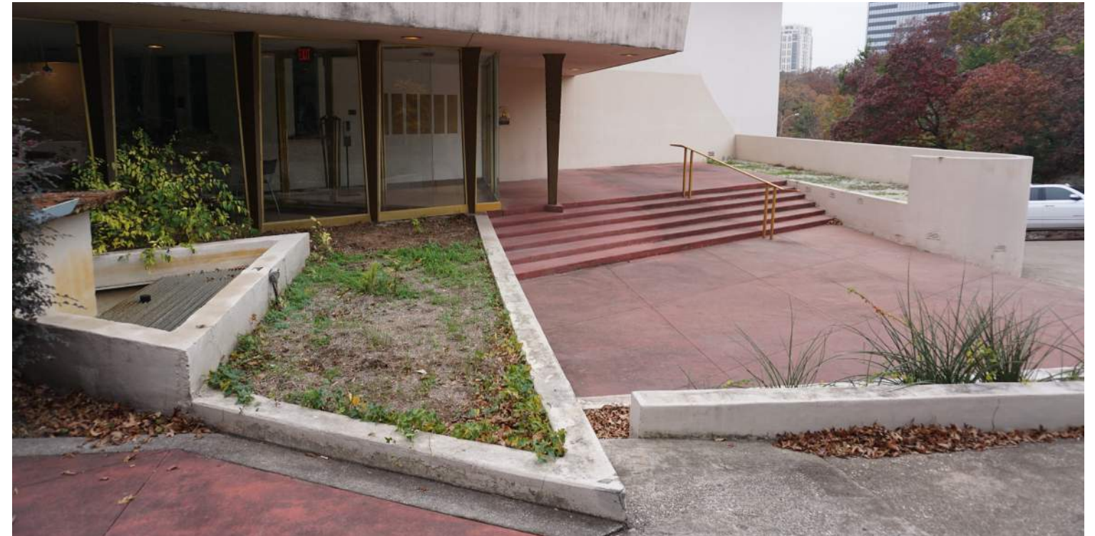
North entry existing condition
