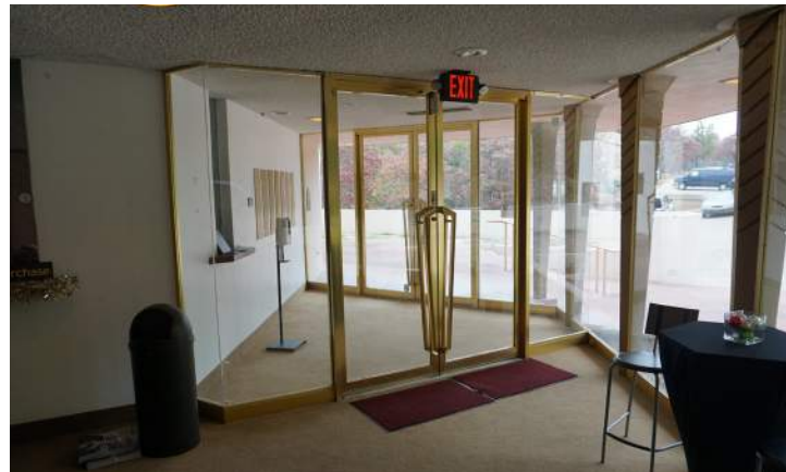
Non-original vestibule with what are believed to be original exterior doors.
