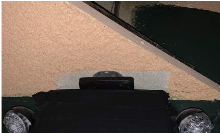
Potentially original finish texture at auditorium ceiling.
