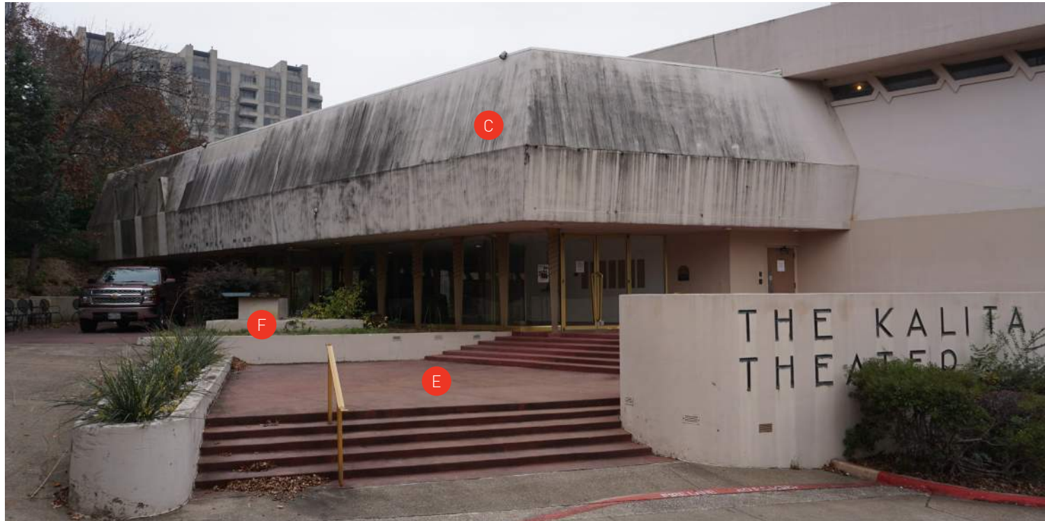
Historic primary entry to Kalita to be restored to 1959 condition.
