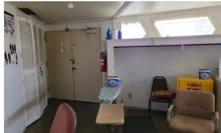
View of plenum level work room.
