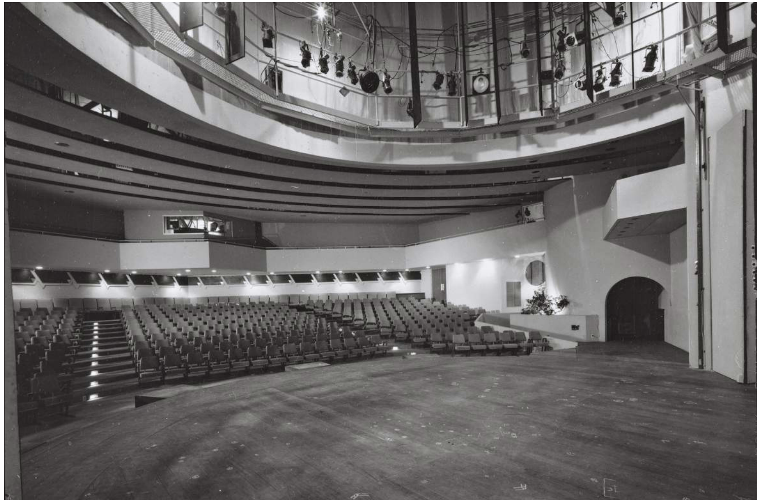
Original condition of the stage circulation to be restored, including restoring the original stage height and dimensions.
