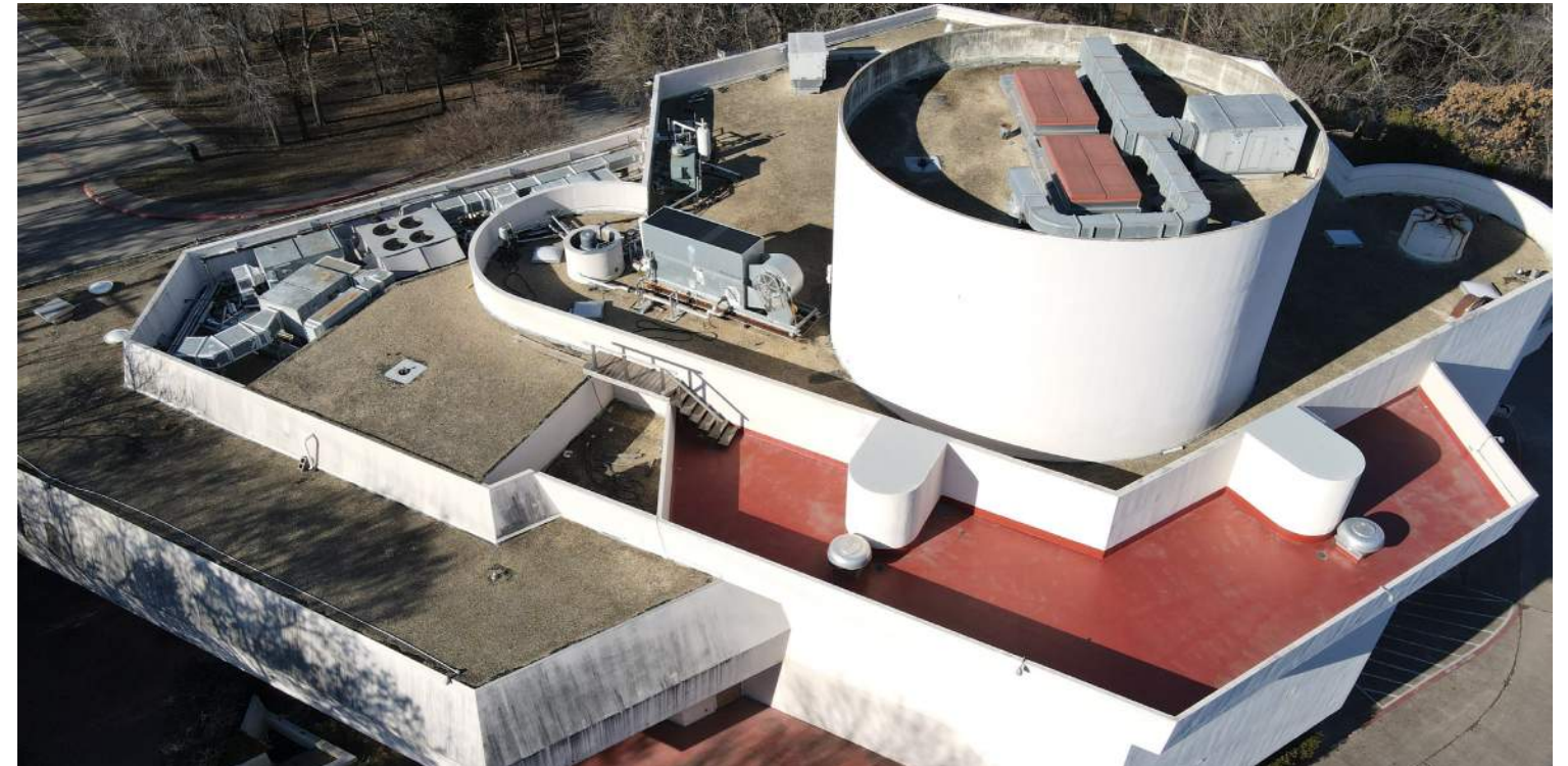
Existing conditions of flat roofs and roof terraces
