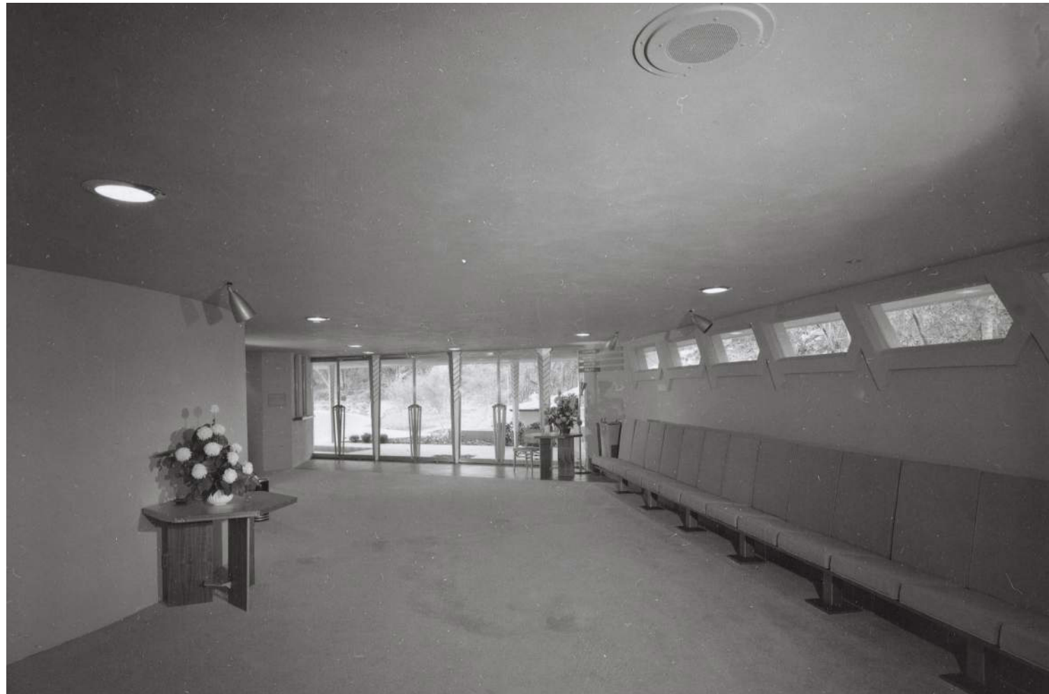
Original condition of lobby with built-in banquette seating to be restored.
