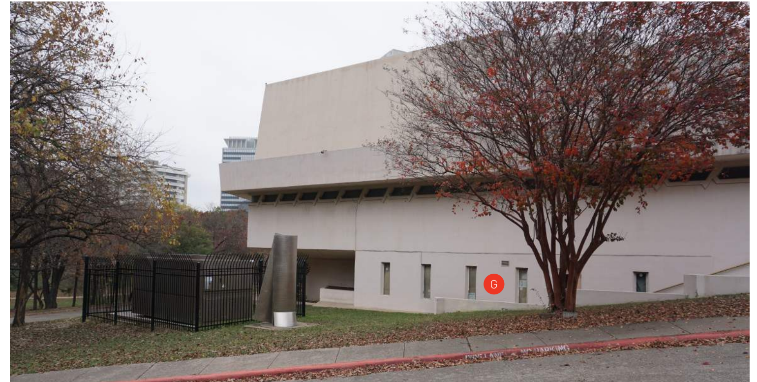
Remove non-original office addition and relocate exterior MEP equipment, refer to MEP recommendations.
