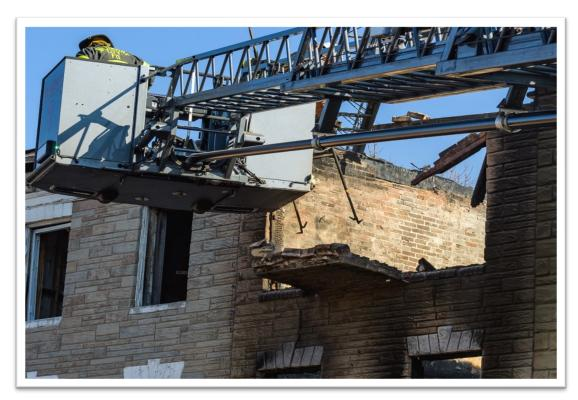
Figure 69 Hooks were used to remove large sections that were cut with saw (Stanley Jaworski)
