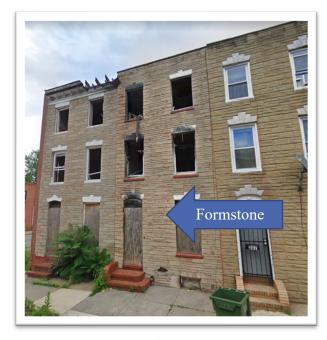
Figure 21 Side Alpha brick façade with a Formstone covering
