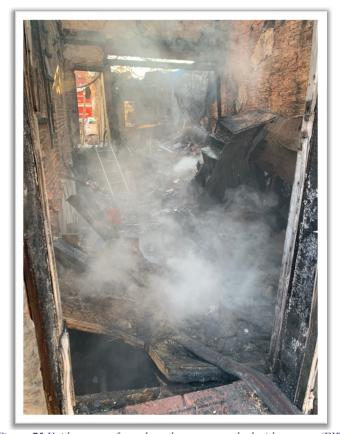
Figure 75 Void space at front door that was searched with camera (FIB)
