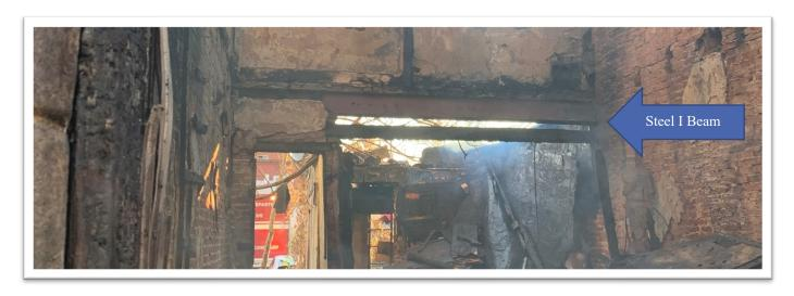
Figure 18 Steel I-beam running across Charlie Side rear wall (FIB)
