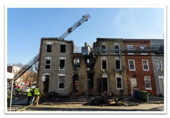
Figure 70 Bricks from third floor Side Alpha have been removed (Stanley Jaworski)
