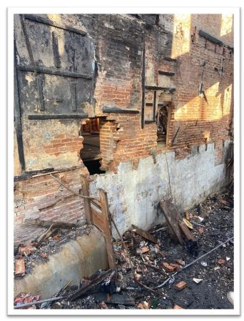
Figure 49 Breaches in the Bravo exposure wall (BCFD Member)
