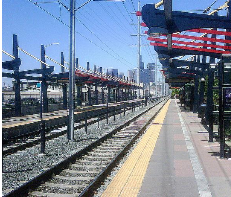
Figure 1. Concrete Tie-and-Ballast Track at the Link SODO Station. 2
