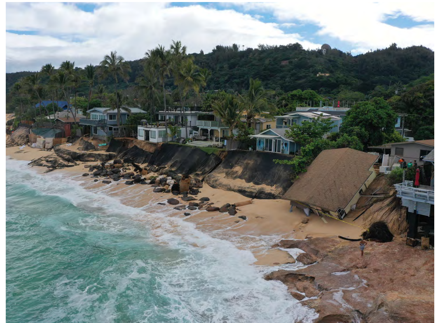
Collapsed home, tarps and other temporary erosion control measures, and impaired beach access between Rocky Point and Sunset Beach Park, North Shore, 2022. Photo: Shellie Habel, Sea Grant/DLNR
