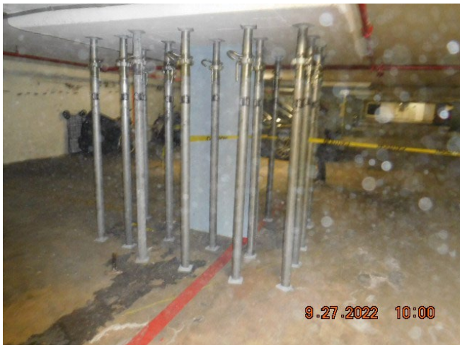
Columns being shored for deck chipping in close proximity and deck spalling.
