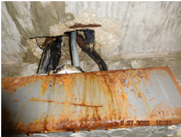
Water leaks into electrical gutter...active
