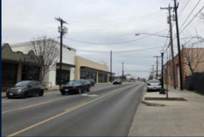
Phase I of the Davis Street Project between Clinton and Beckley was completed in 2020.
