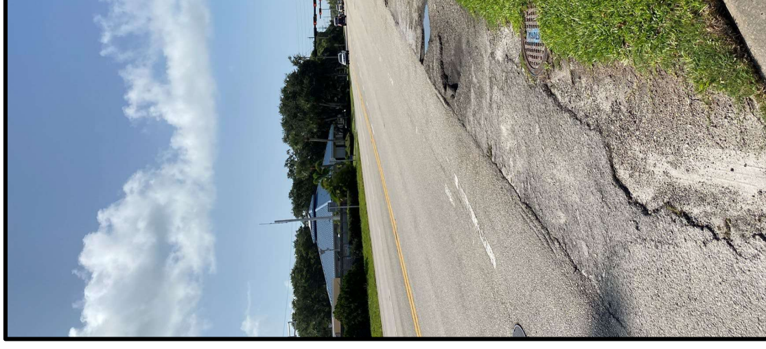
Southbound SR-A1A approach (pre-construct)
