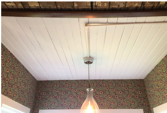
Figure 1-64. Alcove ceiling. (BM, 08/24/2021)
