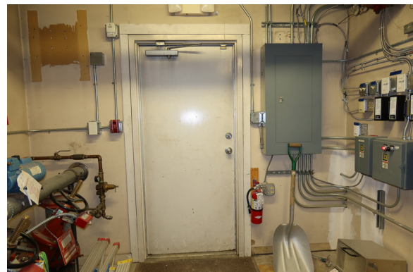
Figure 1-275. South wall of Mechanical Room 110. (EAV, 08/24/2021)
