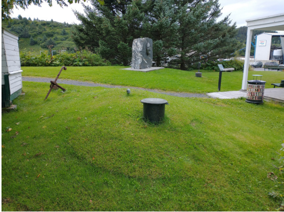
Figure 1-393. Fuel Tank Location (JSW 8/24/2021)
