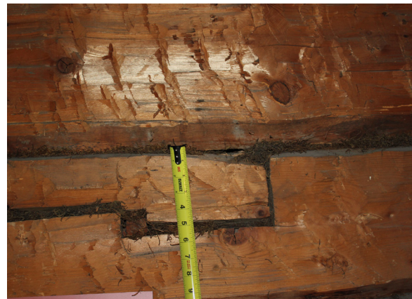
Figure 1-368. Typical log splice found in the first floor walls (CBB, 08/26/2021)
