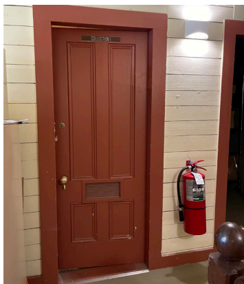
Figure 1-227. Door 201, Stair Hall 200 side. (KAC, 08/24/2021)
