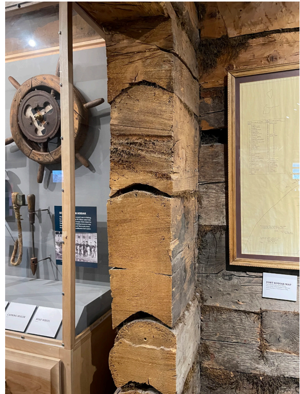
Figure 1-215. Hewn logs and moss chinking at CO 103. (KAC, 08/24/2021)
