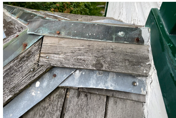
Figure 1-137. Alcove roof and connection to the west facade. (KAC, 08/24/2021)
