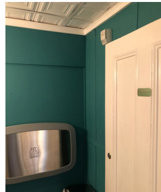
Figure 1-79. Southeast corner and modern ceiling in Restroom 107. (BM, 08/24/2021)
