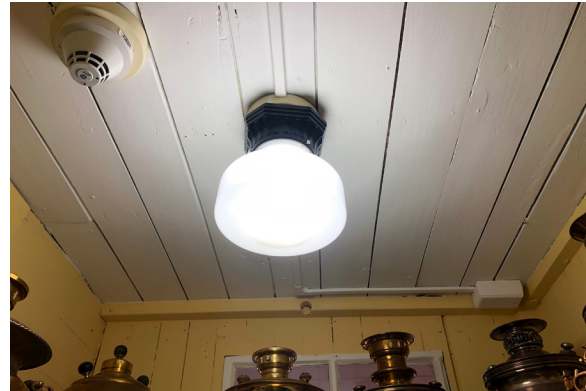
Figure 1-78. Ceiling of Pantry 106. (BM, 08/24/2021)
