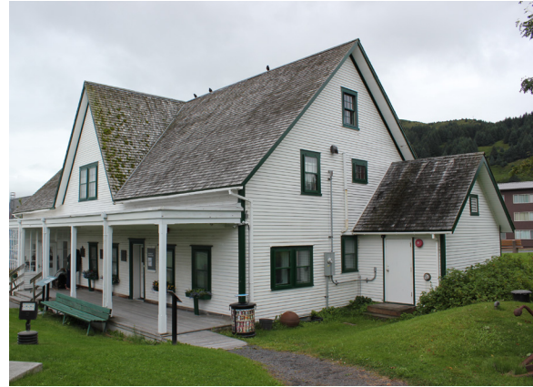
Figure 1-345. Southeast corner of the Russian-American Company Magazin. Note the sun porch on the south elevation and the Mechanical Room addition on the east elevation (CBB, 08/24/2021)
