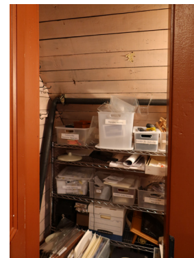
Figure 1-316. Looking south into Storage 205A. (EAV, 08/24/2021)
