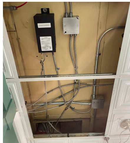
Figure 1-269. Historic ceiling finish above the suspended ceiling in Kitchen 108. (EAV, 08/24/2021)
