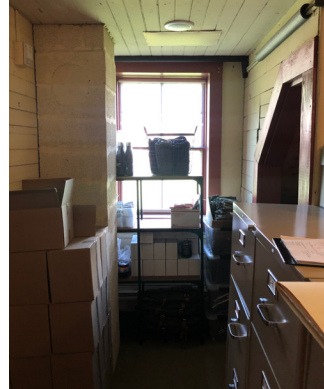
Figure 1-91. Facing north in Stair Hall 200. (BM, 08/24/2021)
