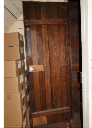
Figure 1-240. Door 300, Attic I 300 side. (EAV, 08/24/2021)
