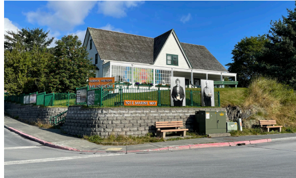
Figure 1-128. Concrete block retaining walls rise along Center Street and East Marine Way (Anderson Hallas, 2021).
