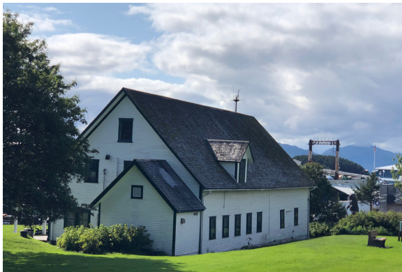
Figure 1-23. Northeast corner of the Magazin, Mechanical Addition in foreground. (BM, 08/24/2021)
