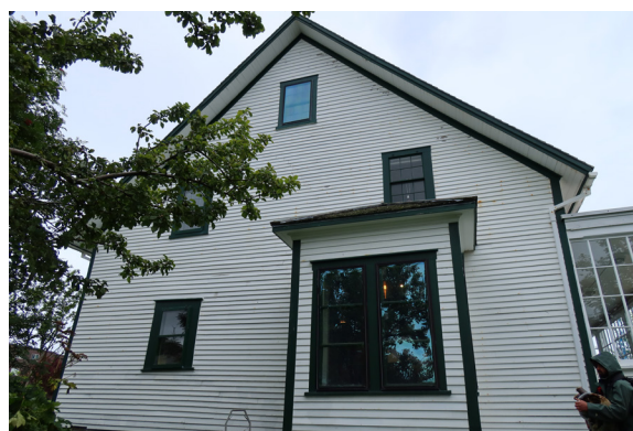
Figure 1-154. West facade. (EAV, 08/24/2021)
