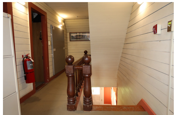
Figure 1-298. Facing south in Stair Hall 200. (EAV, 08/24/2021)
