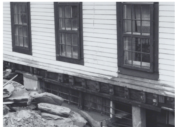
Figure 1-164. Historic storm windows along north facade. (Kodiak History Museum, ca. 1970s)
