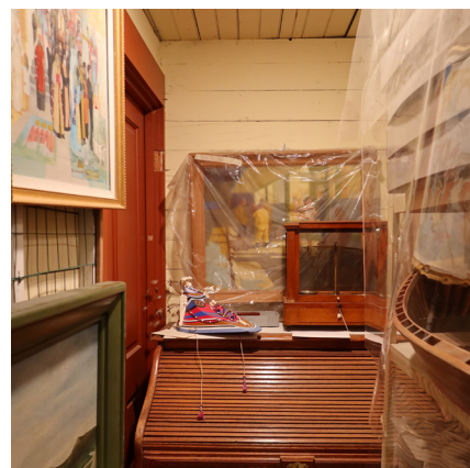
Figure 1-233. Door 203B is blocked by collections in Collections III 203. (EAV, 08/24/2021)
