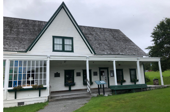
Figure 1-32. South facade, enclosed porch at image left. (BM, 08/24/2021)
