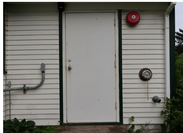
Figure 1-203. Door 110 exterior. (EAV, 08/24/2021)
