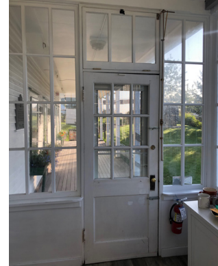
Figure 1-69. East wall of the Sun Porch 103. (BM, 08/24/2021)
