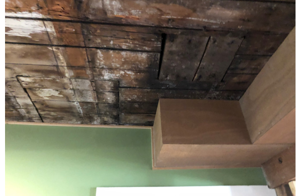
Figure 1-75. Ceiling in Museum II 104. (BM, 08/24/2021)
