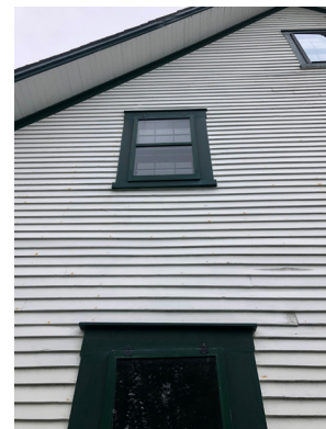
Figure 1-43. Window 29 at image center. (BM, 08/24/2021)
