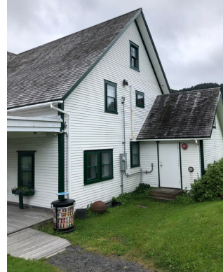
Figure 1-36. Southeast corner, Mechanical Addition at image right. (BM, 08/24/2021)
