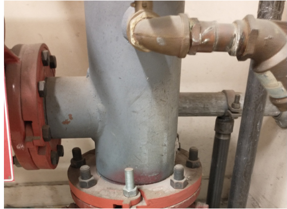
Figure 1-383. Combination Fire and Water Entry (JSW 8/24/2021)
