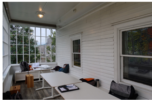
Figure 1-191. Built-in bench in front of Windows 05 and 06. (EAV, 08/24/2021)
