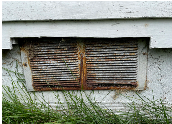
Figure 1-160. Foundation vent and notched siding at the north facade. (KAC, 08/24/2021)
