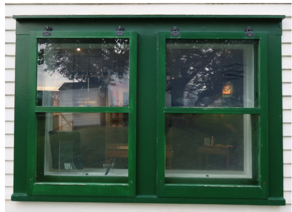
Figure 1-184. Window 26A/B, Type A. (EAV, 08/24/2021)
