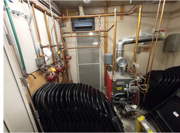
Figure 1-370. Hydronic System (JSW 8/24/2021)
