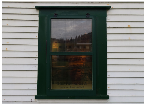
Figure 1-161. Window 22 with typical window trim. (EAV, 08/24/2021)
