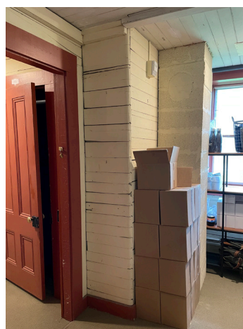
Figure 1-300. Facing northwest in Stair Hall 200. (EAV, 08/24/2021)
