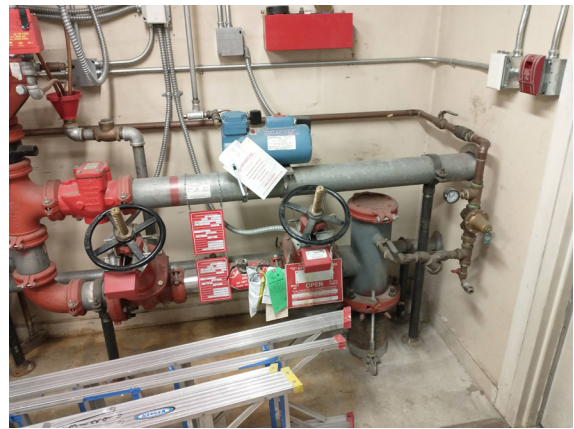
Figure 1-395. Compressor for Dry Pipe Fire Protection (JSW 8/24/2021)
