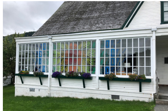
Figure 1-30. South facade of enclosed porch. (BM, 08/24/2021)
