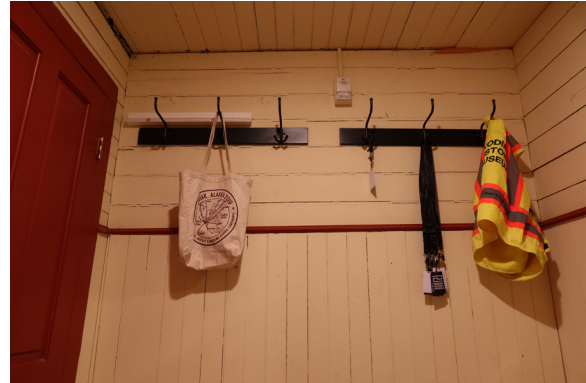
Figure 1-321. West wall of Staff Restroom 207, upper half. (EAV, 08/24/2021)
