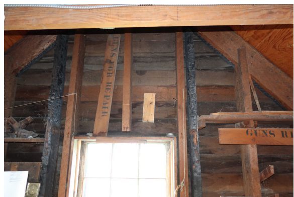
Figure 1-339. West wall of Attic I 300. (EAV, 08/24/2021)
