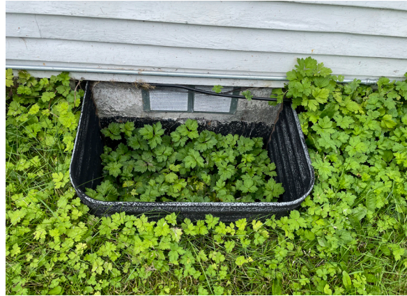
Figure 1-156. Window well on the east elevation. (KAC, 08/24/2021)
