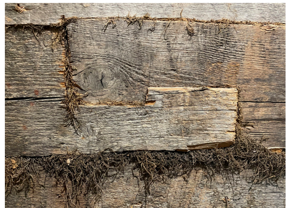
Figure 1-56. Logs with moss chinking and square-notched joint. (KAC, 08/24/2021)
