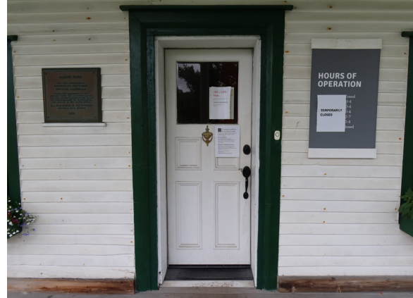
Figure 1-198. Door 100 exterior. (EAV, 08/24/2021)
