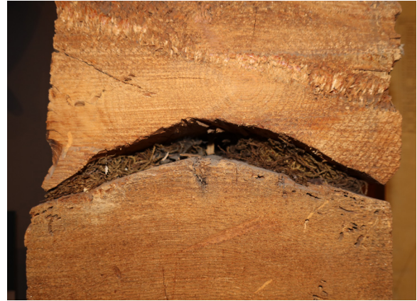
Figure 1-214. Hewn logs and moss chinking at CO 103. (EAV, 08/24/2021)
