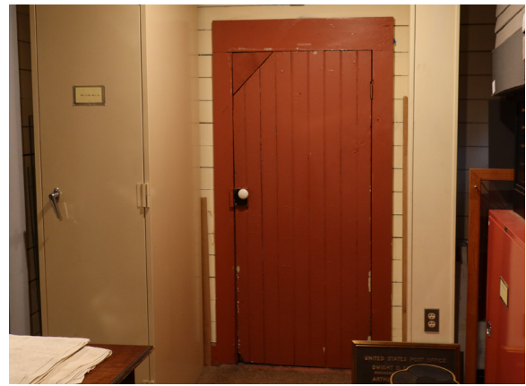
Figure 1-229. Door 201B, Collections I 201 side. (EAV, 08/24/2021)
