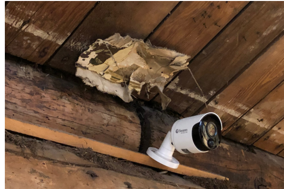
Figure 1-61. Remnants of wallpaper at ceiling. (BM, 08/24/2021)
