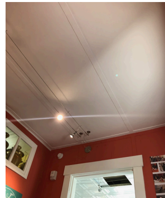
Figure 1-52. Ceiling at Entry 100. (BM, 08/24/2021)
