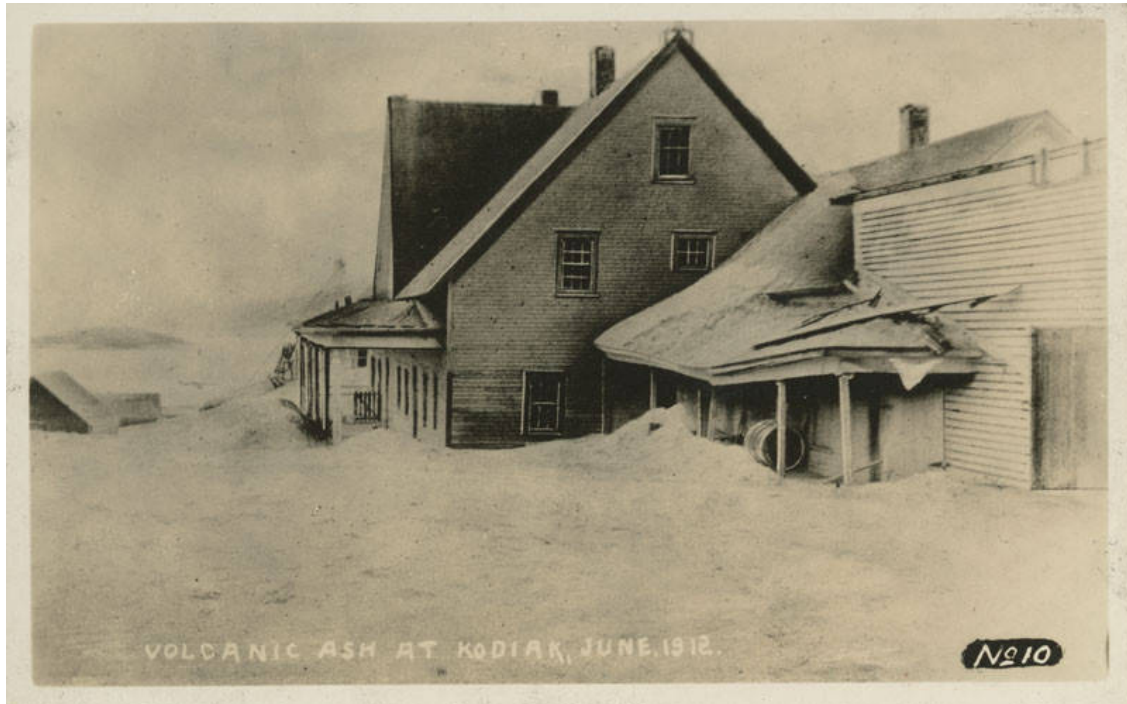
Figure 1-10. 1912 photograph of the deep ash resulting from the Mt. Katmai eruption. This image does not show the low wall at the west end of the porch. (Source: Kodiak Historical Museum, KHM P-368-5-10-a).
