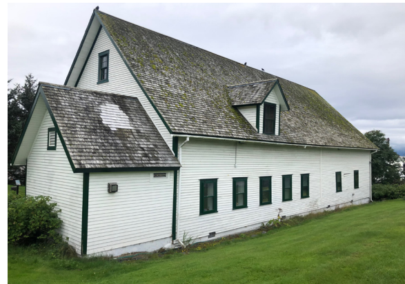
Figure 1-34. Northeast corner. (BM, 08/24/2021)
