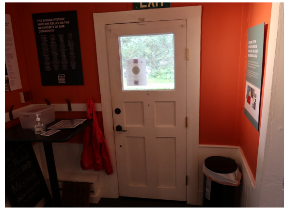
Figure 1-199. Door 100 interior. (EAV, 08/24/2021)
