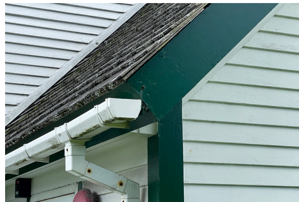
Figure 1-139. Eave condition at the addition showing fascia, gutter, and downspout. (KAC, 08/24/2021)
