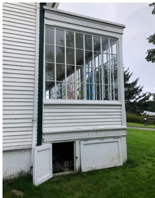
Figure 1-40. West elevation of enclosed porch. (BM, 08/24/2021)
