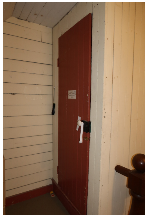
Figure 1-244. Stair Hall 200 side of Door 300. (EAV, 08/24/2021)
