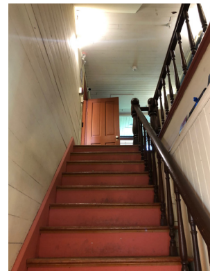
Figure 1-88. Looking up the stairs to the second floor. (BM, 08/24/2021)
