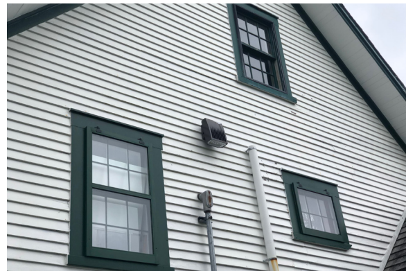
Figure 1-38. Second and third floor windows at west facade. (BM, 08/24/2021)
