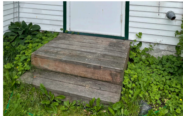
Figure 1-148. Stoop at the mechanical addition. (KAC, 08/24/2021)
