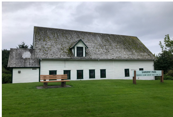
Figure 1-35. North facade. (BM, 08/24/2021)
