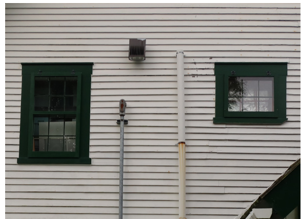
Figure 1-188. Right to left: Windows 31 and 32, Type E and D. (EAV, 08/24/2021)
