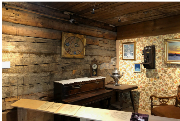
Figure 1-60. New partition wall in Museum I 102 abuts the historic log wall. (BM, 08/24/2021)
