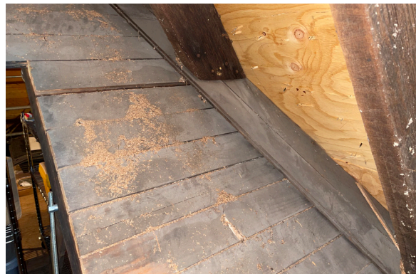
Figure 1-342. Sheathing with cut access hole, Attic II 301 side. (KAC, 08/24/2021)
