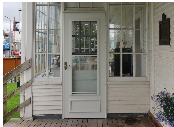
Figure 1-200. Door 103B exterior. (EAV, 08/24/2021)
