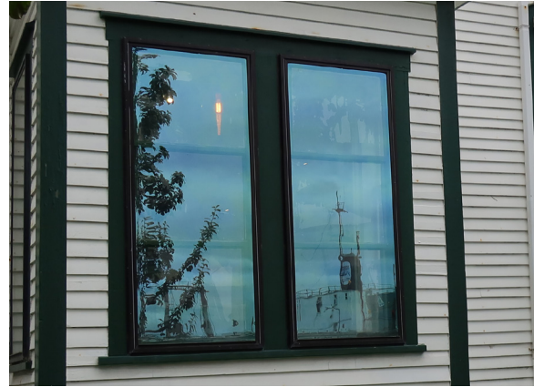
Figure 1-173. Windows 14 and 15, Type B. (EAV, 08/24/2021)
