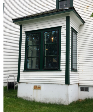
Figure 1-41. West elevation of alcove. (BM, 08/24/2021)
