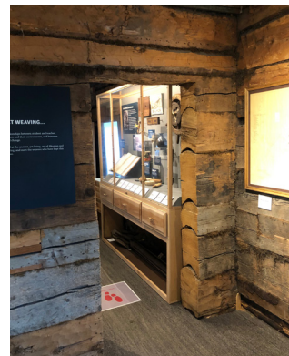
Figure 1-71. Facing west at CO 103. (BM, 08/24/2021)
