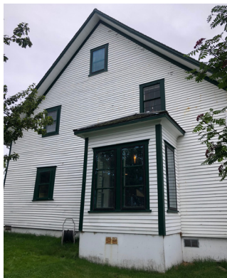
Figure 1-24. West facade, alcove in foreground. (BM, 08/24/2021)
