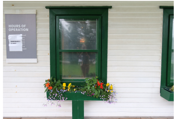
Figure 1-162. Trim with mitered corners and window box at Window 02, Type A. (EAV, 08/24/2021)
