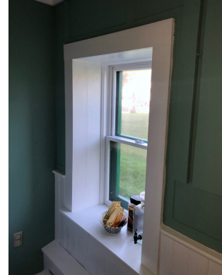
Figure 1-84. Window at north wall of Staff Kitchen 109. (BM, 08/24/2021)
