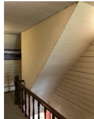
Figure 1-92. Facing southwest in Stair Hall 200. (BM, 08/24/2021)
