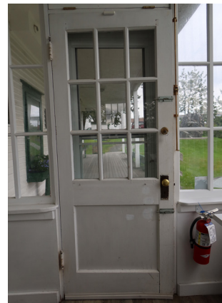
Figure 1-202. Door 103B interior. (EAV, 08/24/2021)
