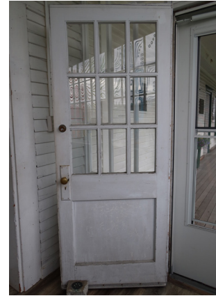
Figure 1-201. Door 103B exterior side of interior panel. (EAV, 08/24/2021)
