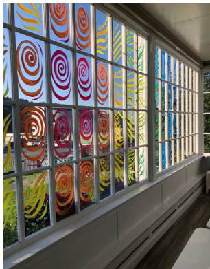
Figure 1-68. South wall of the Sun Porch 103. (BM, 08/24/2021)
