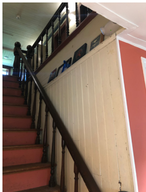
Figure 1-90. East wall adjacent to the stairs to the second floor. (BM, 08/24/2021)
