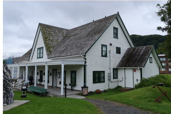
Figure 1-135. Magazin viewed from southeast. The primary gable roof, large dormer, mechanical addition, and porch are visible here. (EAV, 08/24/2021)
