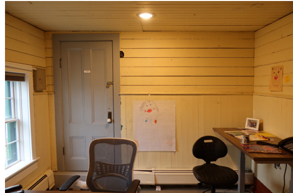
Figure 1-324. North wall of Director's Office 208. (EAV, 08/24/2021).
