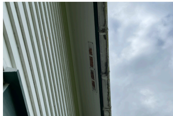
Figure 1-140. Enclosed eave with fixed louver vent. (KAC, 08/24/2021)
