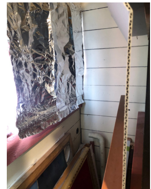
Figure 1-96. Window 31 at interior. (BM, 08/24/2021)
