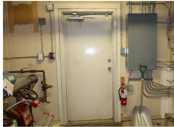
Figure 1-204. Door 110 interior. (EAV, 08/24/2021)
