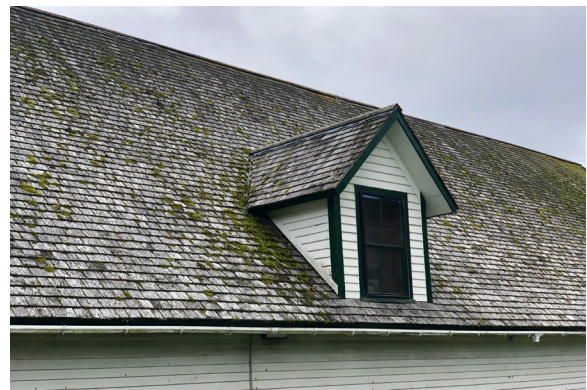
Figure 1-26. Small roof dormer at north facade. (BM, 08/24/2021)
