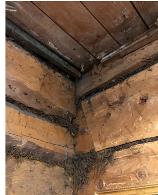
Figure 1-45. Historic log wall dividing interior spaces on the first floor. (BM, 08/24/2021)
