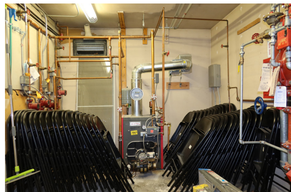
Figure 1-276. North wall of Mechanical Room 110. (EAV, 08/24/2021)
