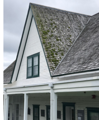
Figure 1-25. Large roof dormer at south facade. (BM, 08/24/2021)
