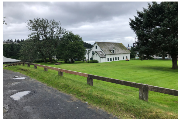
Figure 1-21. Magazin viewed from east access drive. (BM, 08/24/2021)
