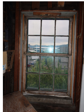
Figure 1-196. Window 33, interior. (EAV, 08/24/2021)
