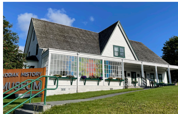
Figure 1-126. Concrete steps and walkway to primary entrance (Anderson Hallas, 2021).
