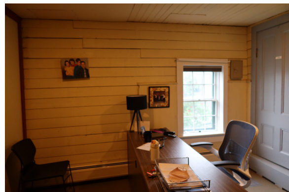
Figure 1-323. West wall of Director's Office 208. (EAV, 08/24/2021)
