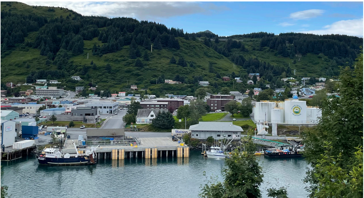
Figure 1-132. The Magazin retains its prominent location on the rise overlooking the harbor (Anderson Hallas, 2021)
