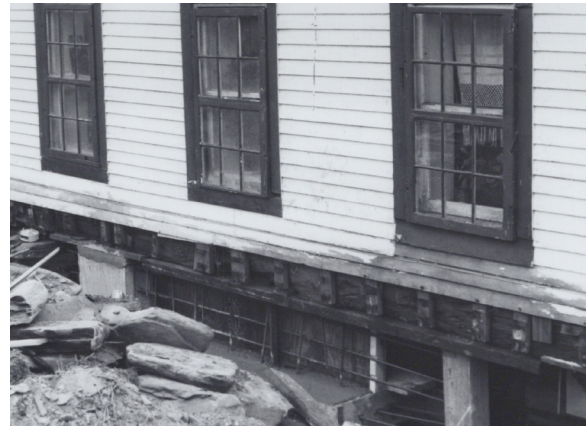
Figure 5-1. Historic twelve-lite storm windows along north facade. (Kodiak History Museum, ca. 1970s)
