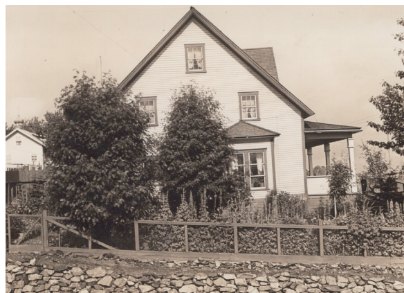
Figure 1-130. Historic wall and perimeter fence (Kodiak Historical Society P-467-26).
