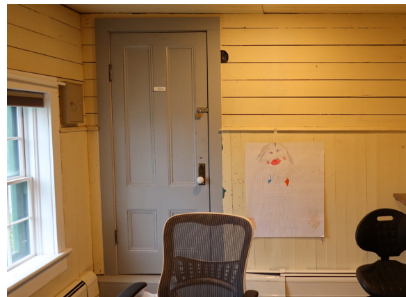
Figure 1-239. Door 208A, Director's Office 208 side. (EAV, 08/24/2021)
