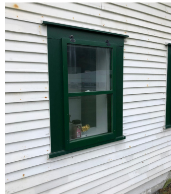
Figure 1-27. Typical first floor window with historically compatible storm. (BM, 08/24/2021)
