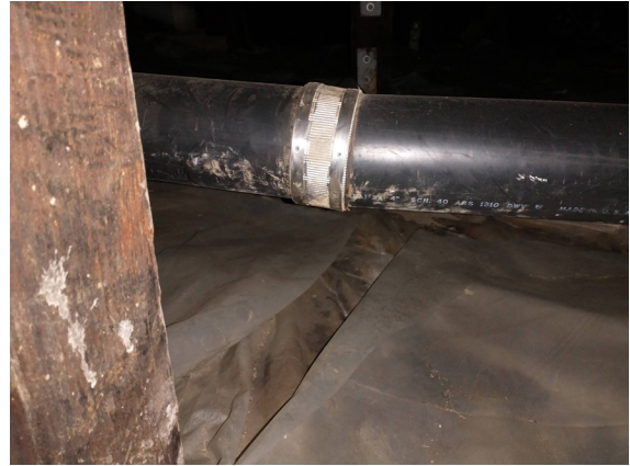
Figure 1-386. ABS Piping in Crawlspace (JSW 8/24/2021)
