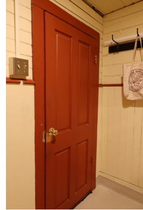
Figure 1-237. Door 207, Staff Restroom 207 side. (EAV, 08/24/2021)
