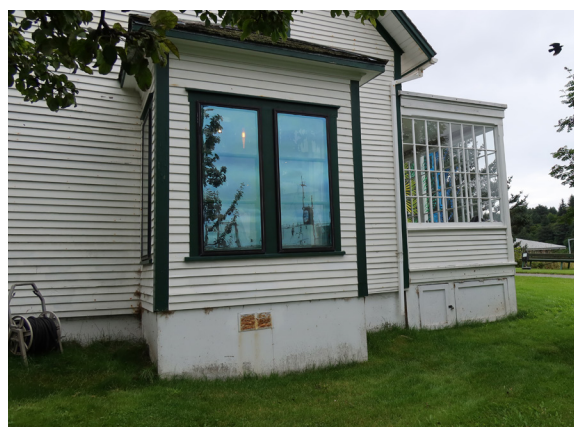
Figure 1-155. Alcove and sun porch viewed from the west. (EAV, 08/24/2021)
