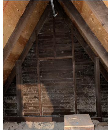
Figure 1-341. South wall of Attic II 302. (EAV, 08/24/2021)
