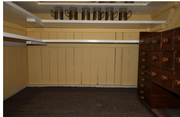
Figure 1-265. Base of south wall of Pantry 106. (EAV, 08/24/2021)
