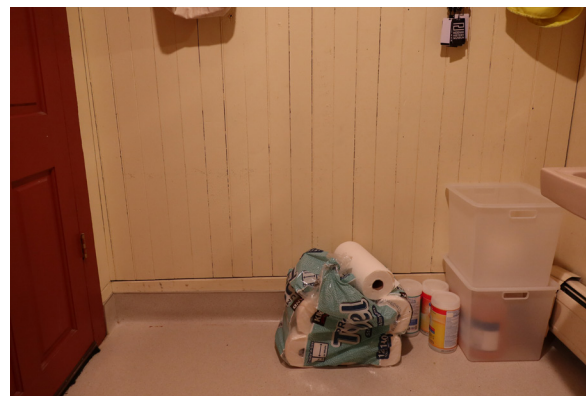
Figure 1-322. Lapped wall base at west wall of Staff Restroom 207. (EAV, 08/24/2021)
