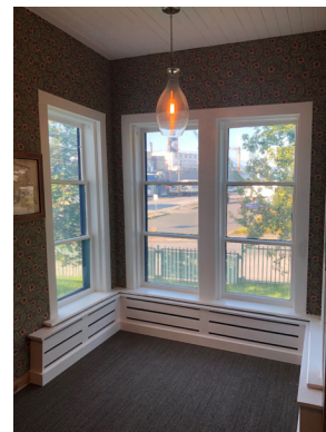
Figure 1-62. Facing west towards the alcove. (BM, 08/24/2021)
