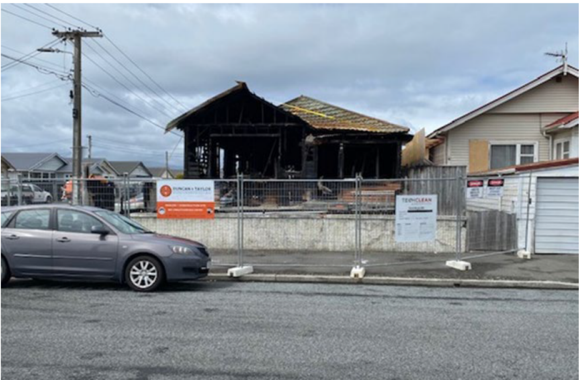
Figure 8 91 Yule Street on 02/03/2022 as seen by the investigation team, one-month post-incident.
