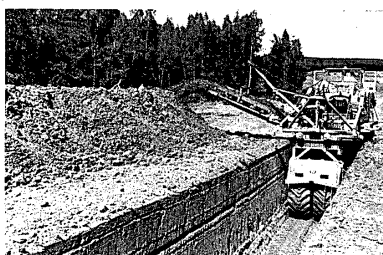
Soviet-made excavator being used to dig pipeline trench.
