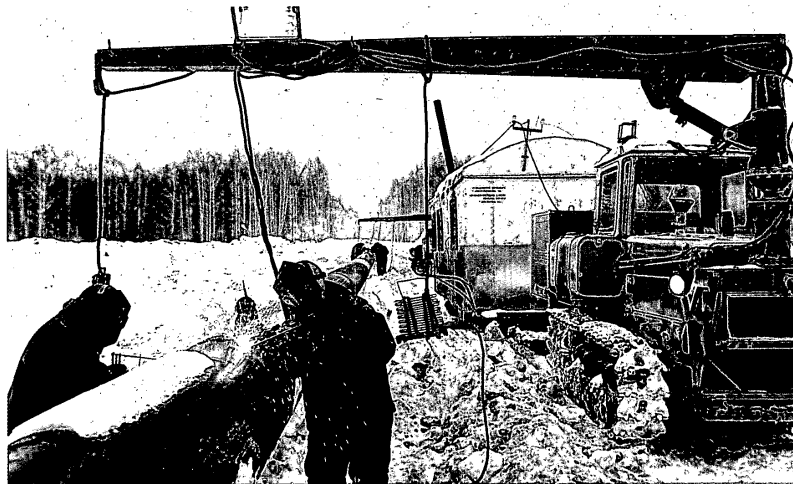
Pipe is welded at storage area welding bases along the pipeline by crews using either manual arc techniques or semiautomatic units.
