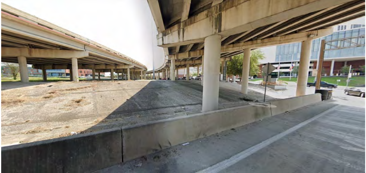
Highway Understory – Existing condition near White Oak Bayou at UHD
