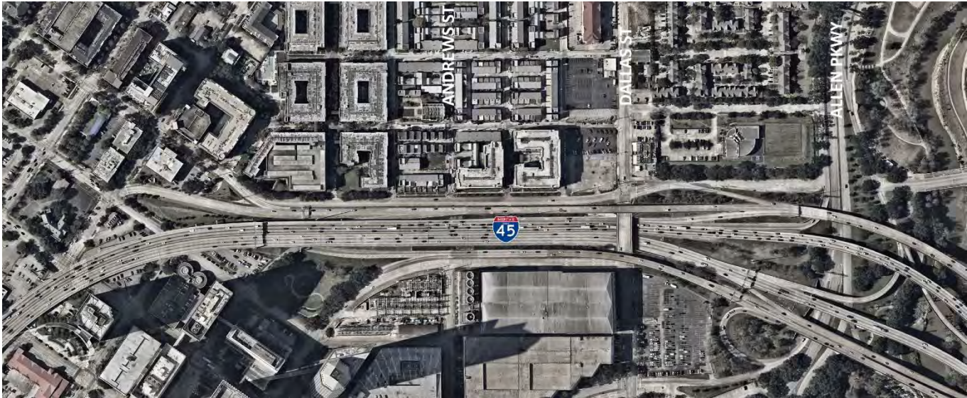
Existing elevated highway cutting off Andrews St
