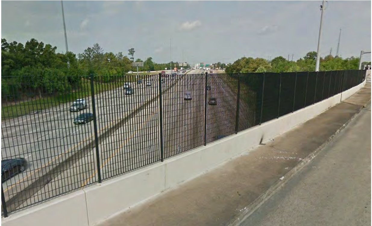
Typical 4'-6' pedestrian realm on street bridge over I-10
