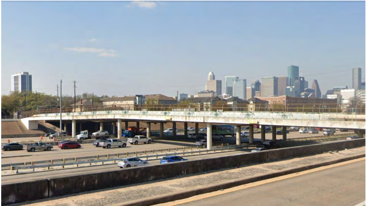
Existing Elgin St Bridge over I-69
