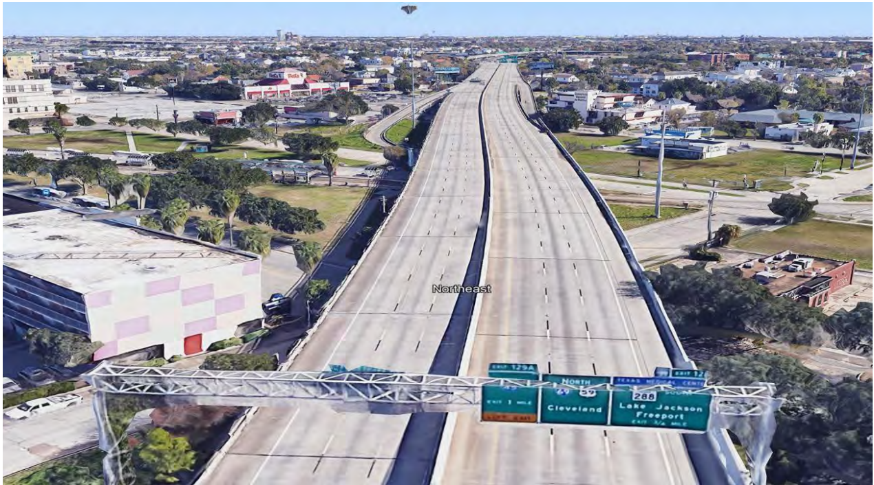
Existing elevated I-69 at Main St
