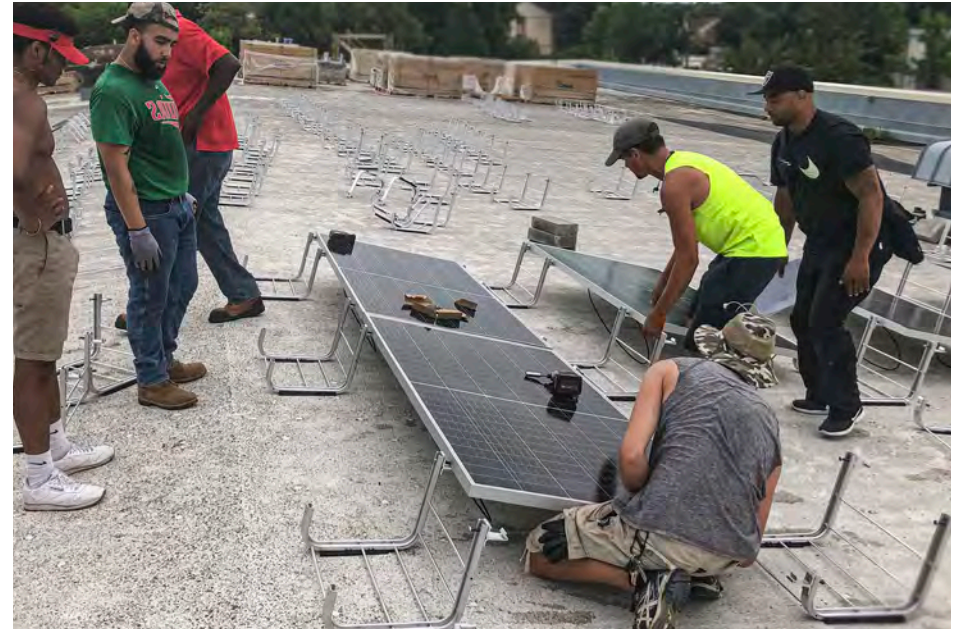
Renewable Energy Partners in Minneapolis does solar installation and skill training in an underserved part of the city.
