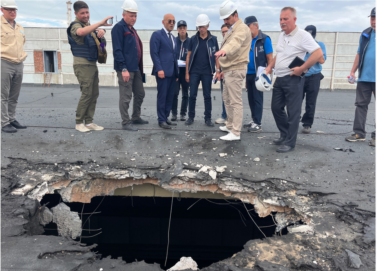
The IAEA team observes the damage caused by shelling on the roof of the special building at the ZNPP that houses, among other items, the fresh nuclear fuel and the solid radioactive waste storage facility. (Photo: IAEA)
