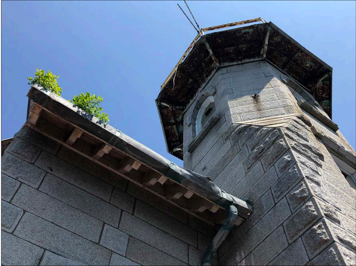
Photo 11. View up the west wall of the Tower and adjoining west eave. Coursed ashlar granite walls remain in extraordinary condition – a testament to their underlying technology – though the assembly possesses several Achilles’ heels: gutters, unpainted cast iron and marginally maintained windows.
