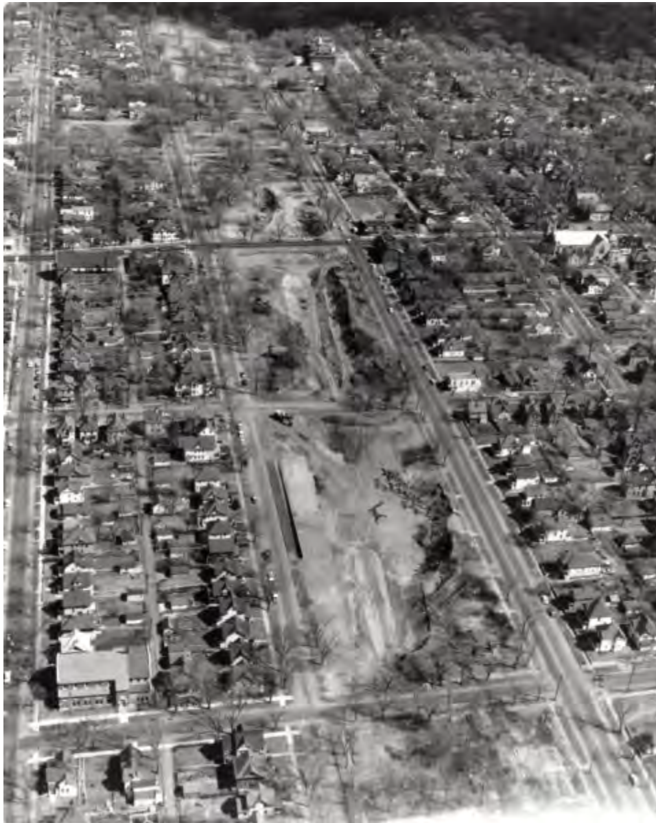
Demolition of homes for construction of I-94 through Rondo
