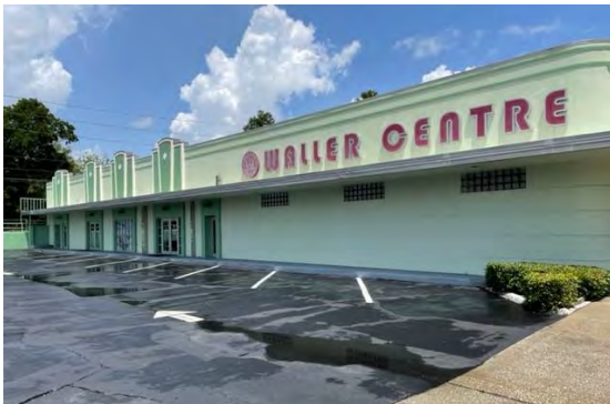
Waller Center and parking at Park St.
