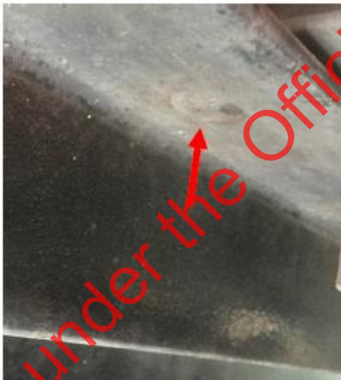
A hint of rust bleed is visible at some joints where the welds are broken, but this is not a reliable method of identifying this problem.
