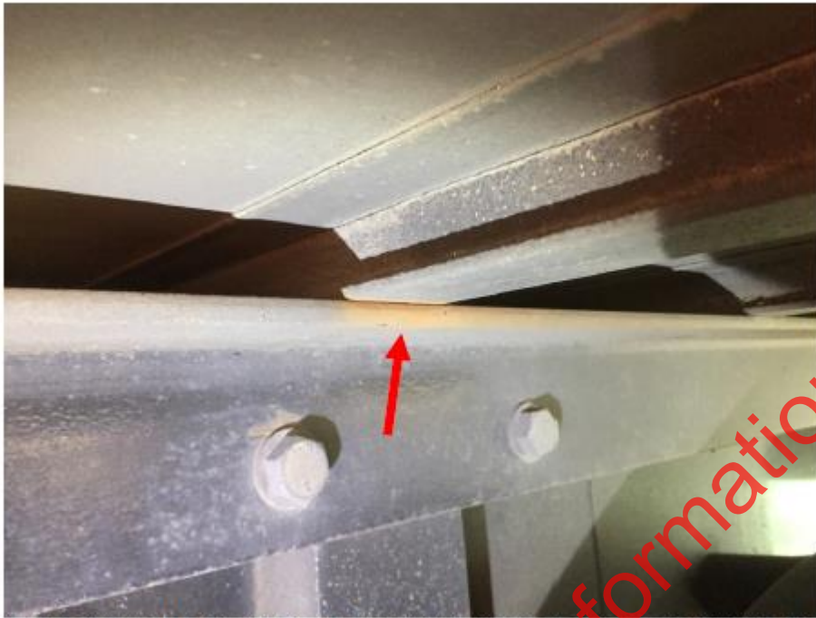
A hint of rust bleed is visible at some joints where the welds are broken, but this is not a reliable method of identifying this problem.
