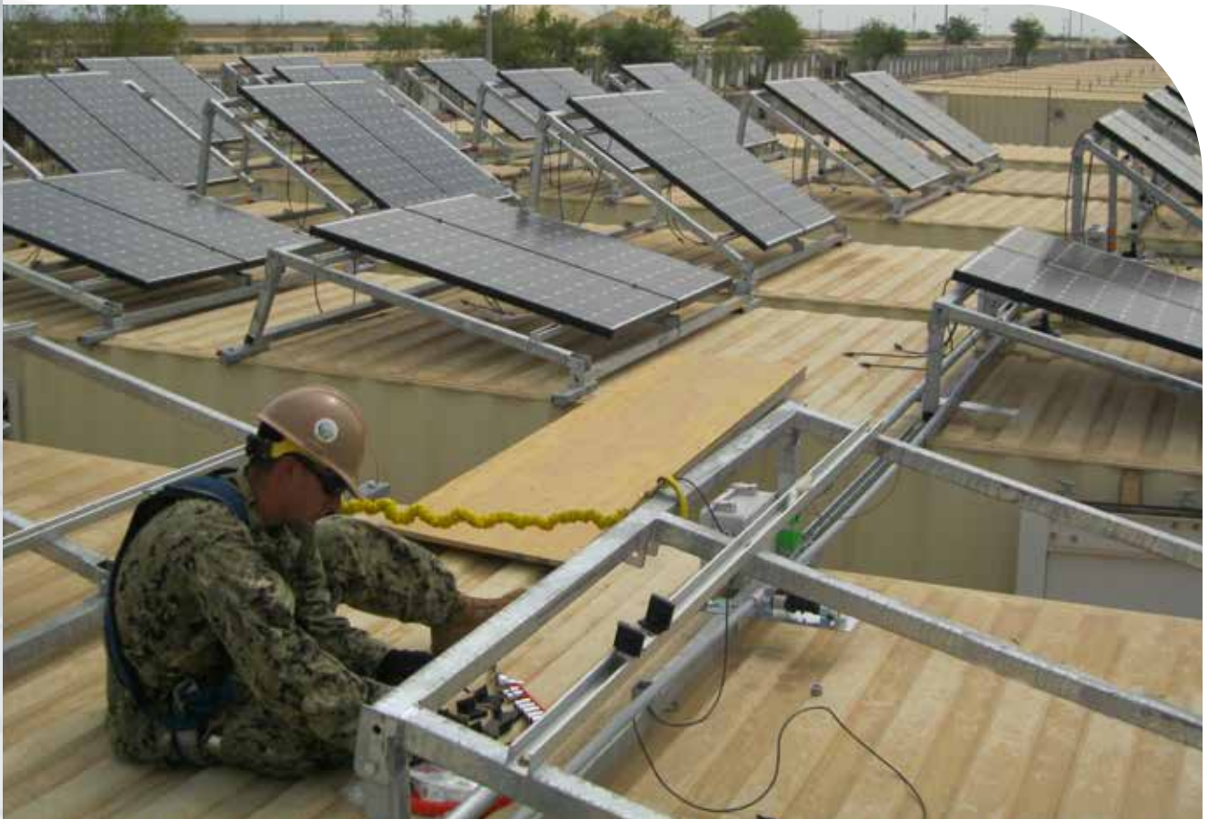
A Sailor with Naval Mobile Construction Battalion 1 (NMCB1) installs a water wash valve atop a containerized living unit at Camp Lemonnier in Djibouti, Africa. NMCB1 installed the arrays to study how the impacts of wind and dust affect the arrays' effectiveness. Solar arrays reduce the base's electrical load and the amount of diesel fuel used to power generators, Sept. 12, 2012.
