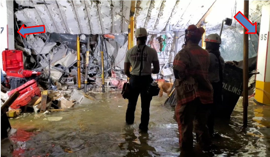
Image 1: Rescue Crew operating between parking columns 95 and 118
