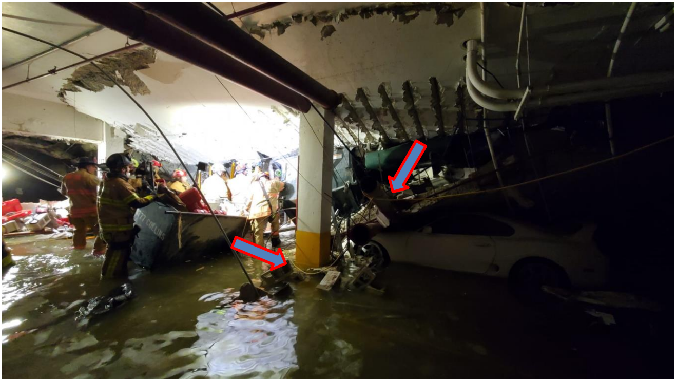
Image 3 - Electrical cords were daisy-chained
